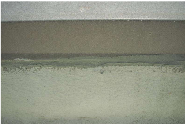
Sealed wall joint.
