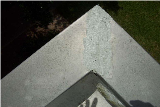
Sealed coping joint.
