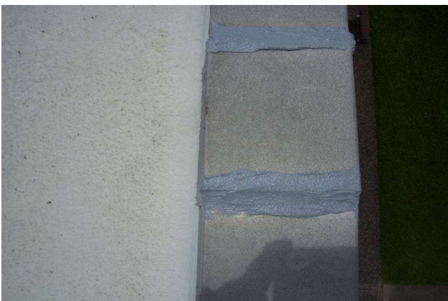
Sealed wall joints.
