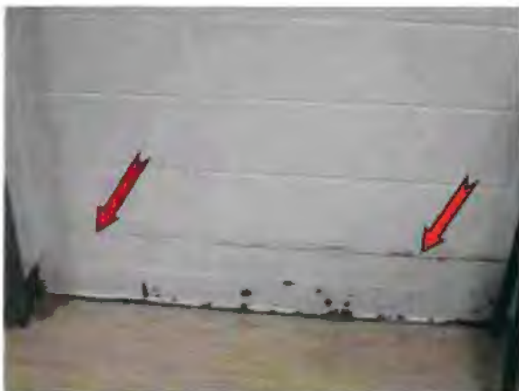
Photo #29 Joint crack in concrete masonry unit wall
