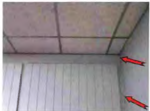
Photo #30 Crack at corner of concrete masonry unit walls
