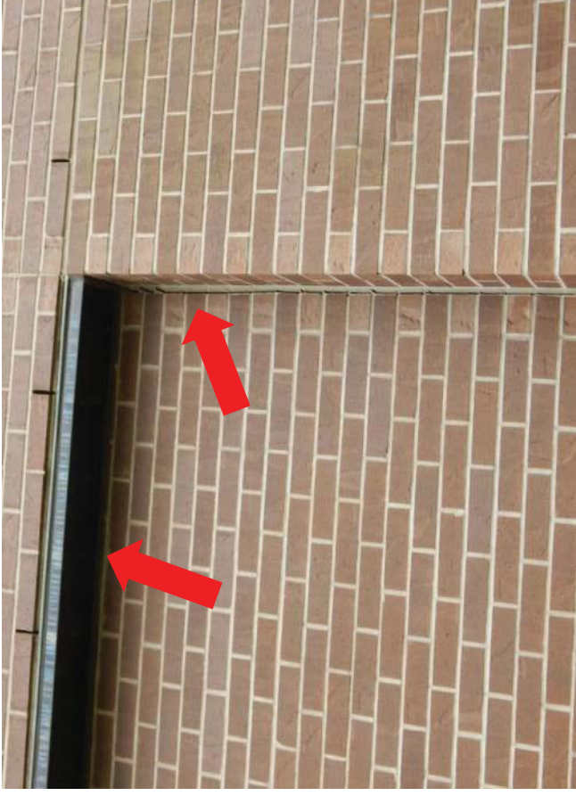
#2 Minor separation in caulk joint at end of inset brick panel. No brick header per architect's detail.
