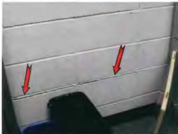
Photo #27 Joint crack in concrete masonry unit wall
