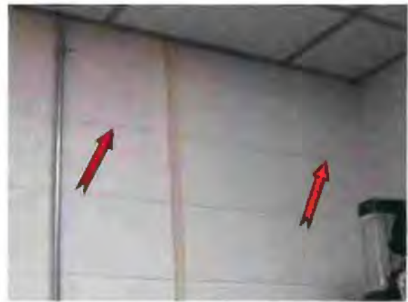
Photo #28 Joint crack in concrete masonry unit wall
