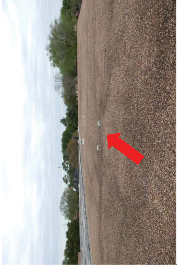
#53 Roof over phase two of community center showing roof drain and emergency drain
