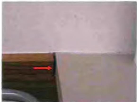
Photo #70 Separation between wood trim and counter top
