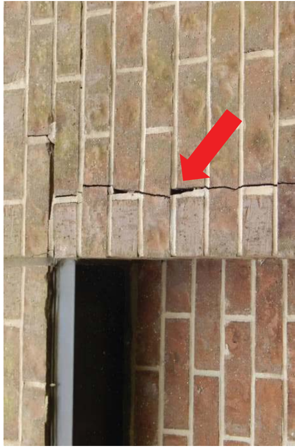
#10 Same as photo #9 at bottom of crack repair and separation in caulk joint.
