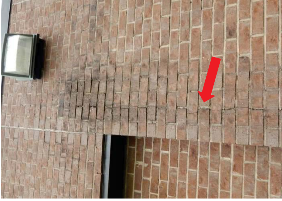
#32 Vertical crack in column brick the same as described in photo #30
