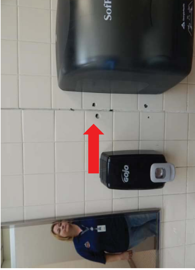
#36 Cracking and movement in tile joint. Mrs. Crenshaw said towel dispenser had to be moved.
