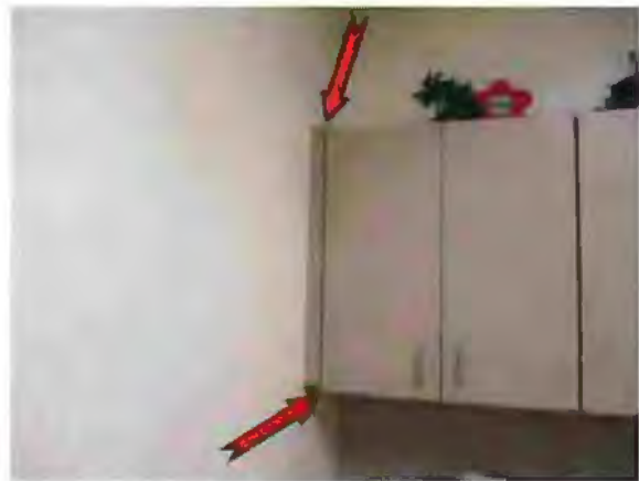
Photo #62 Cabinet doors out-of-square with respect to their frame
