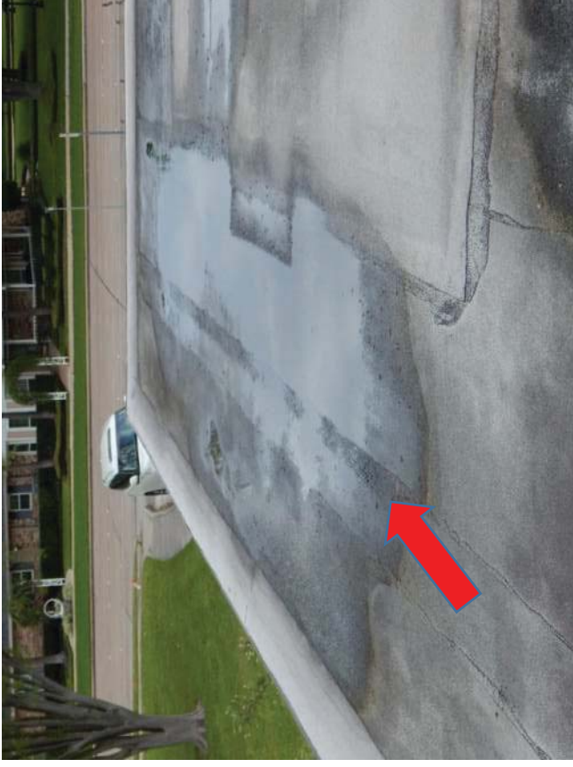
#51 Roof over phase one of community center showing standing water
