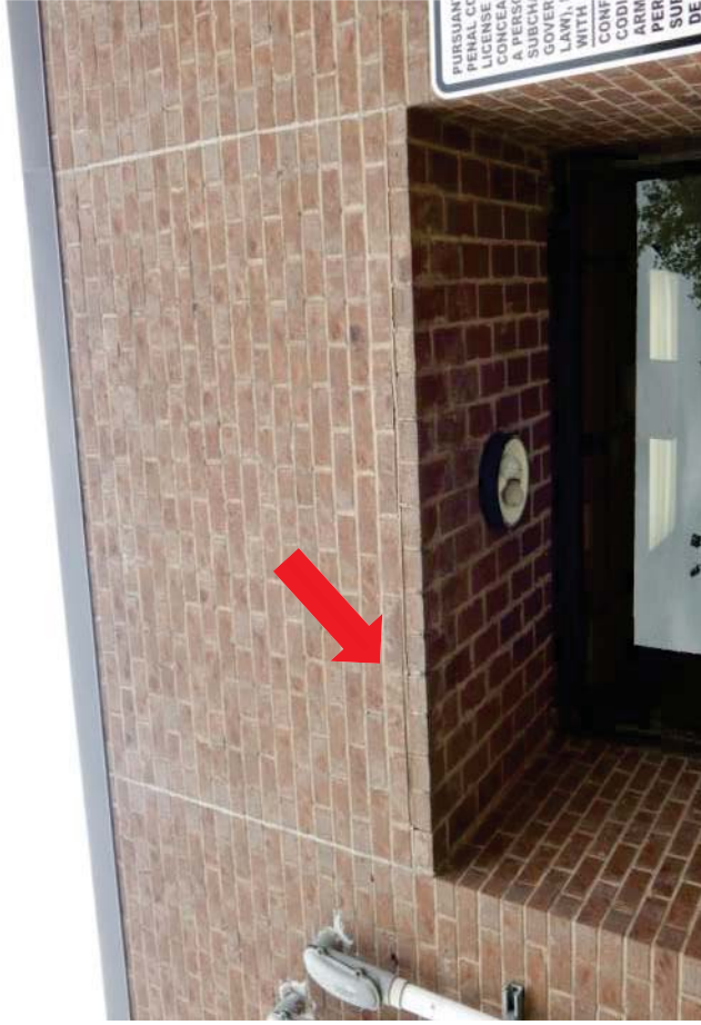
#31 Horizontal crack above soffit brick The same as described in photo #13
