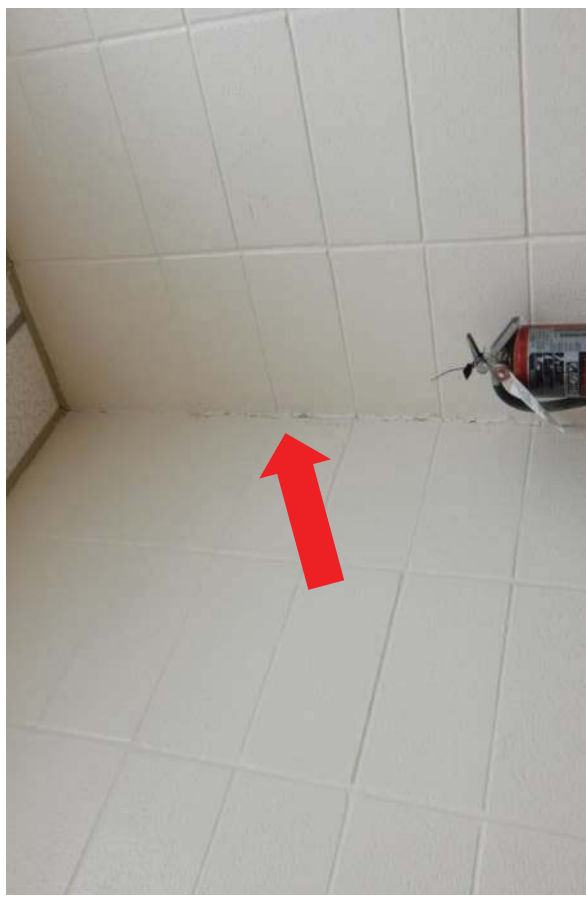
#43 Level on floor showing sloping down toward the North East corner at approximately 1/8" per foot
