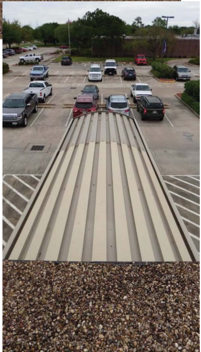
Addition canopy from above
