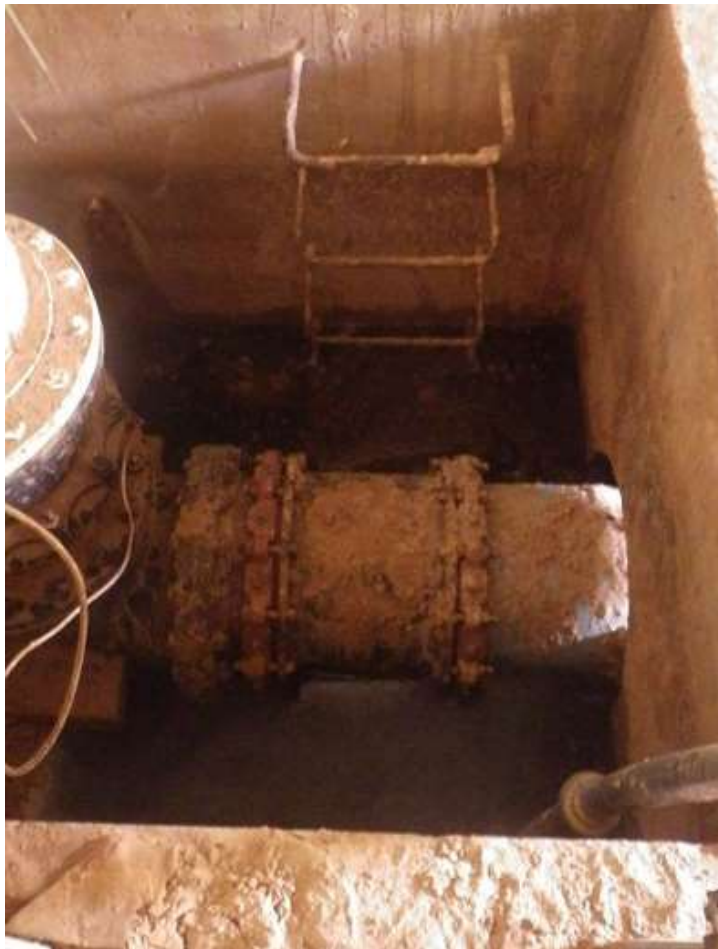
55. Inlet/outlet pipe extending from pipe pit in the base cone floor.
