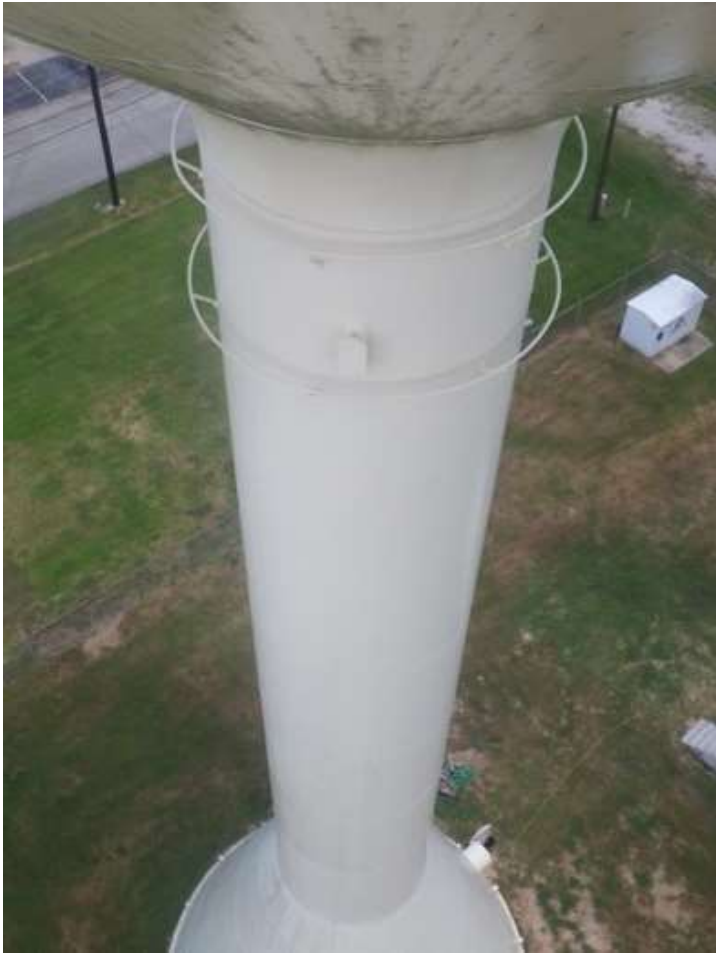
17. Support column, painter's manhole, and painter's rings.
