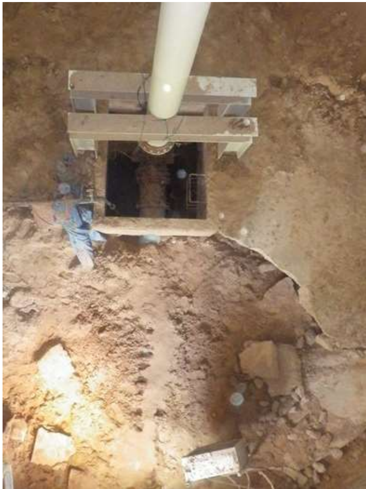
59. Inlet/outlet pipe and brackets.
