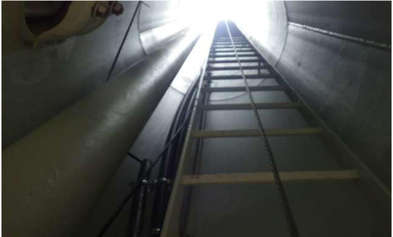
80. Interior dry access tube ladder, safe-climbing device, cables, and overflow pipe.
