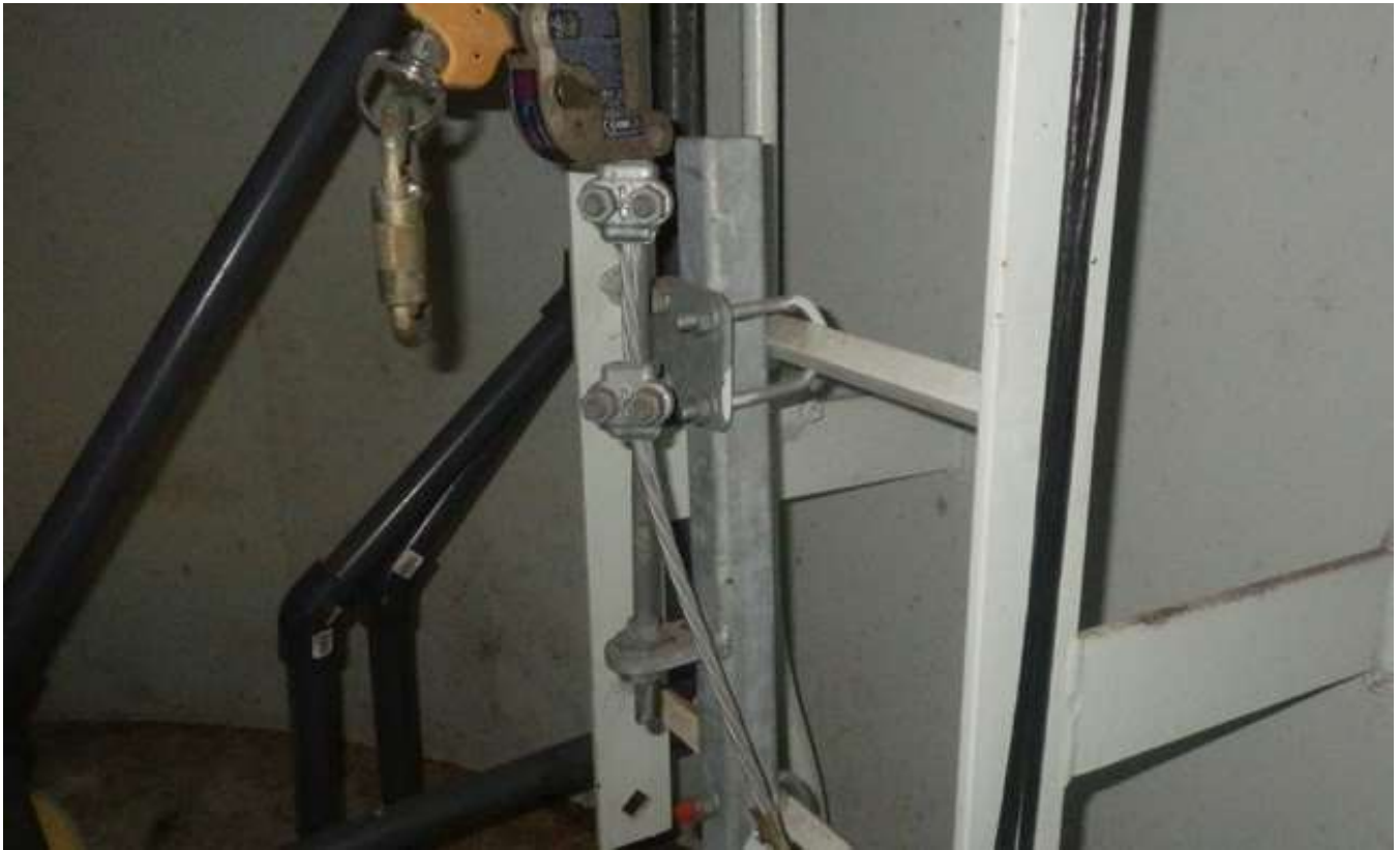
69. Support column ladder, safe-climbing device, and cables.
