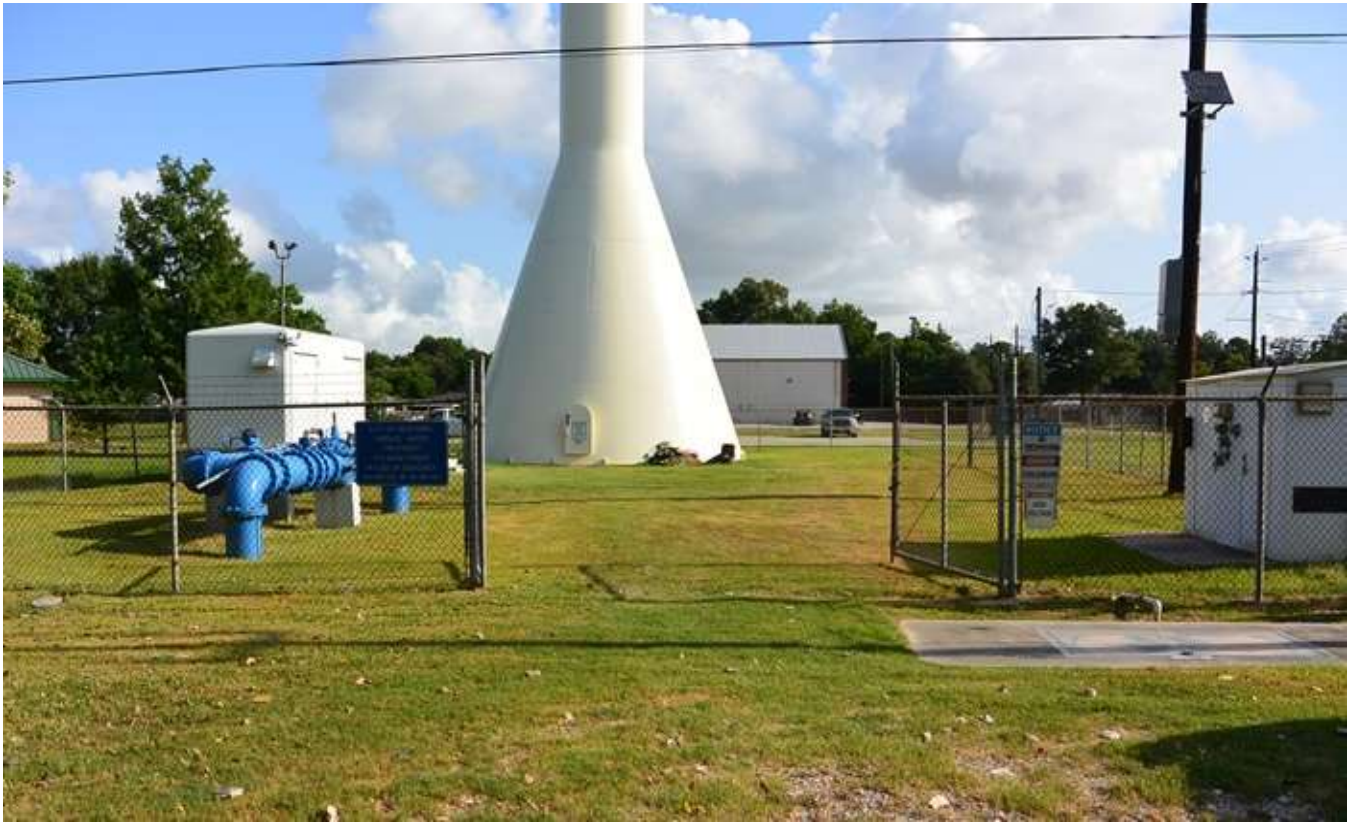
5. Site gate. Note information and warning signs on the fence.
