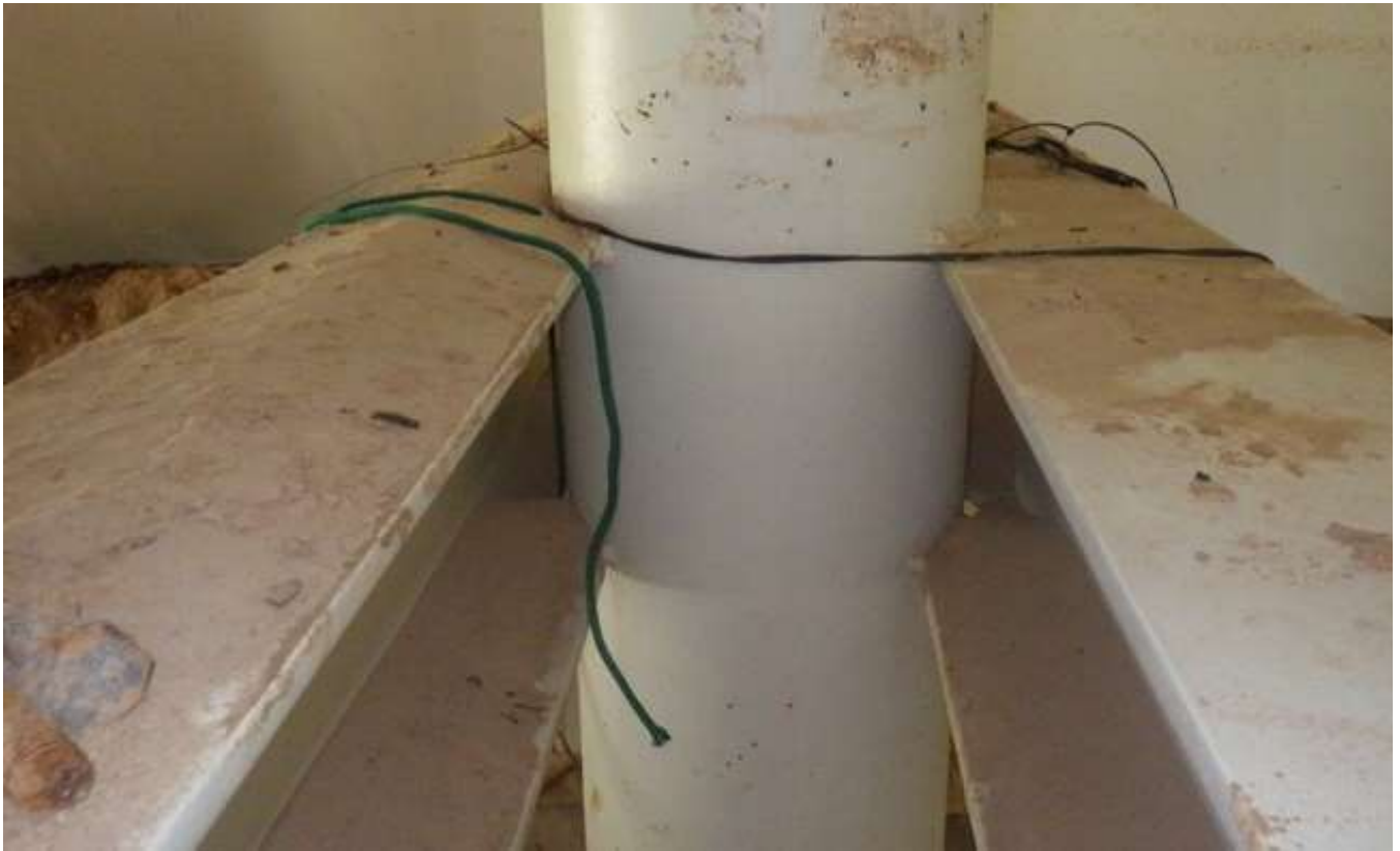
59. Inlet/outlet pipe and brackets.
