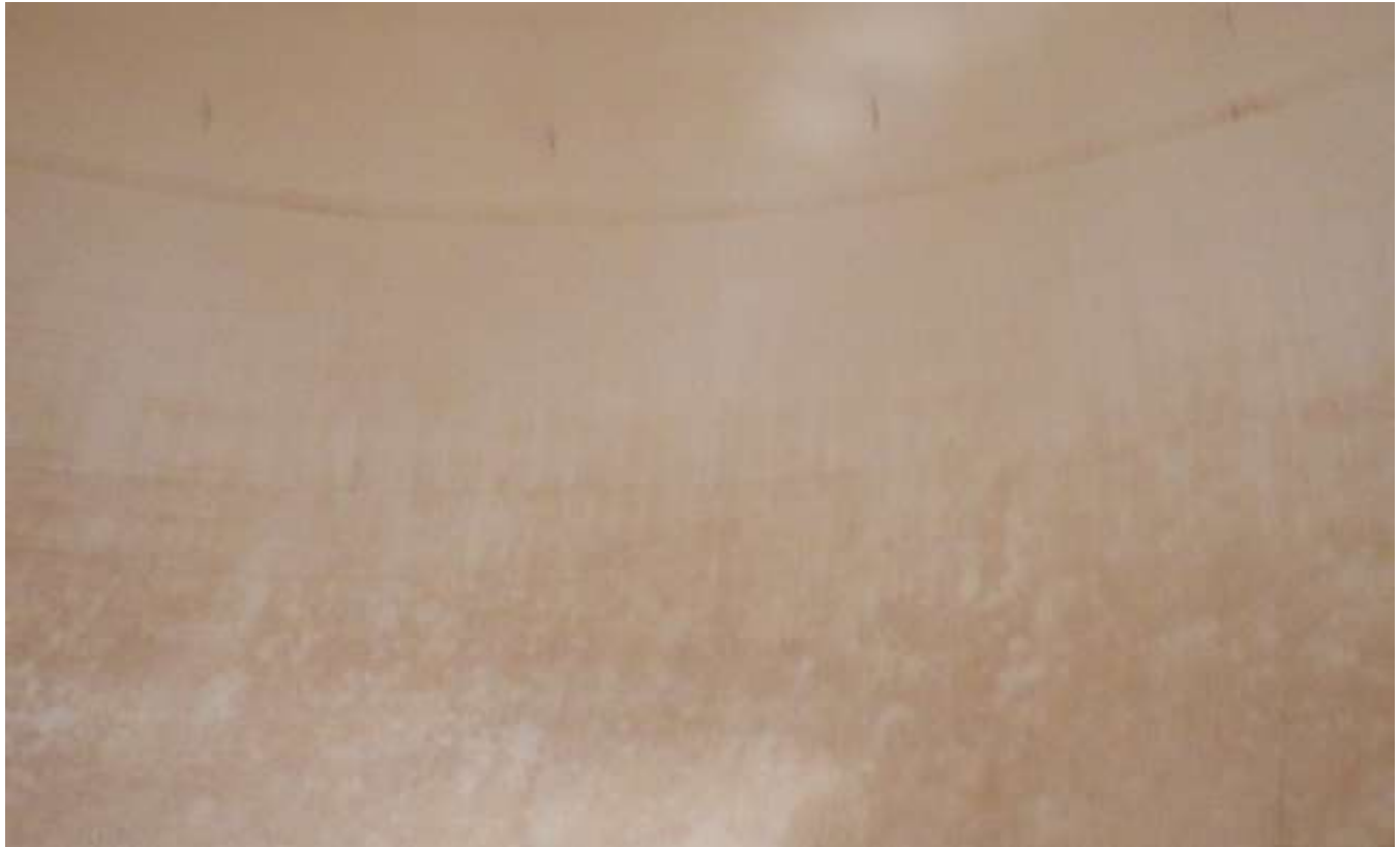
90. Roof and shell interior.
