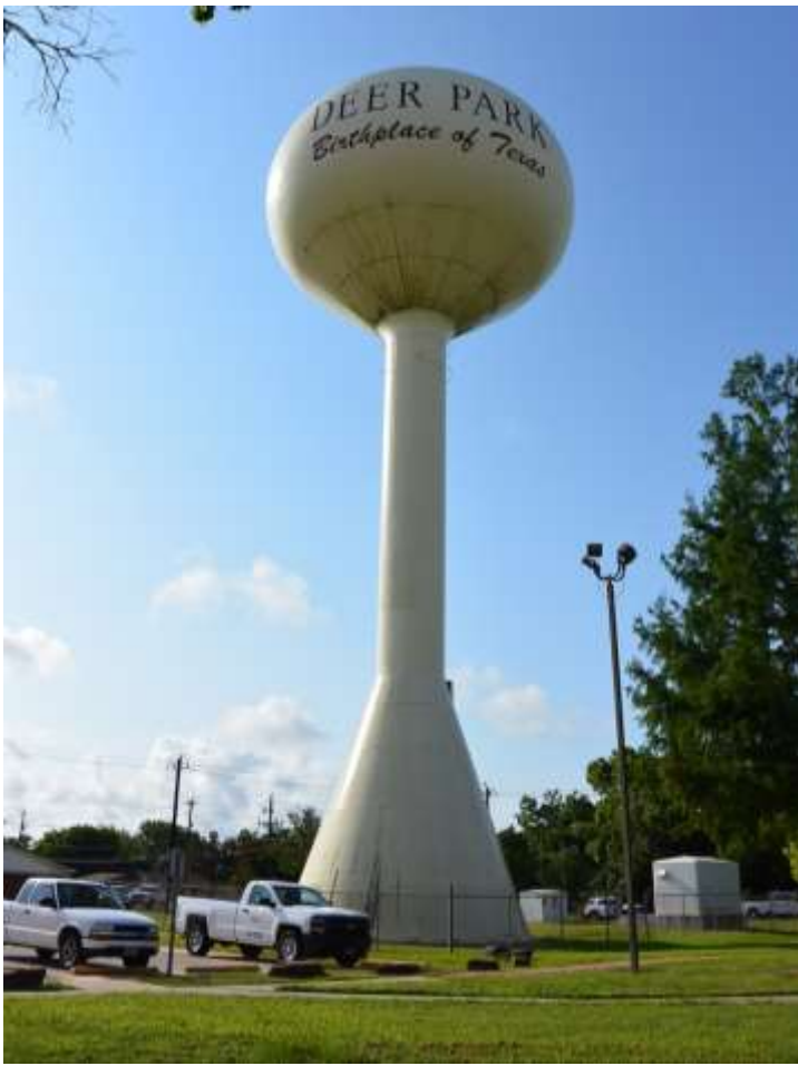
1. Tank and site.
