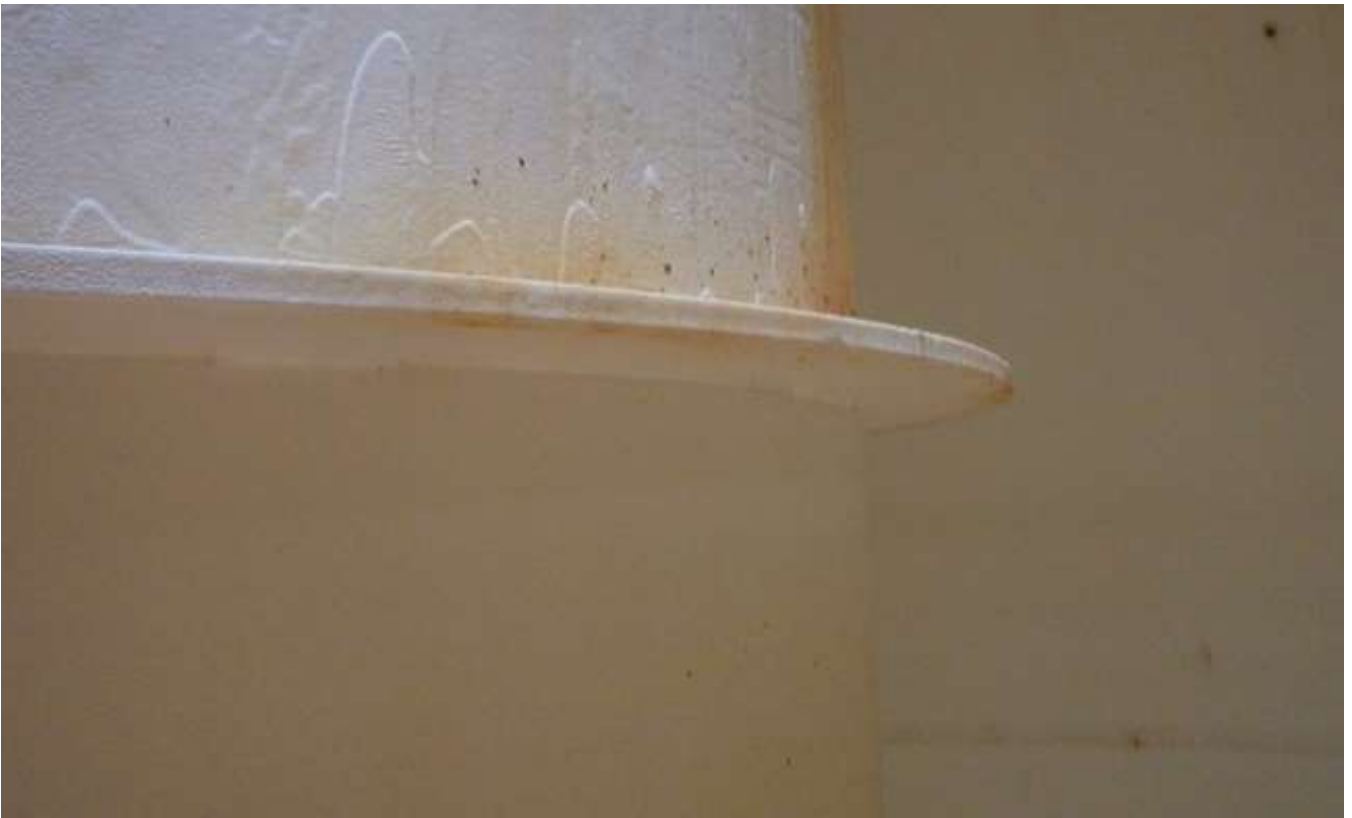
96. Interior wet access tube stiffener.
