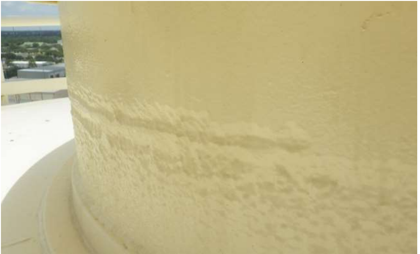
39. Pitting which had occurred prior to the last repainting on the access tube roof manhole curb.
