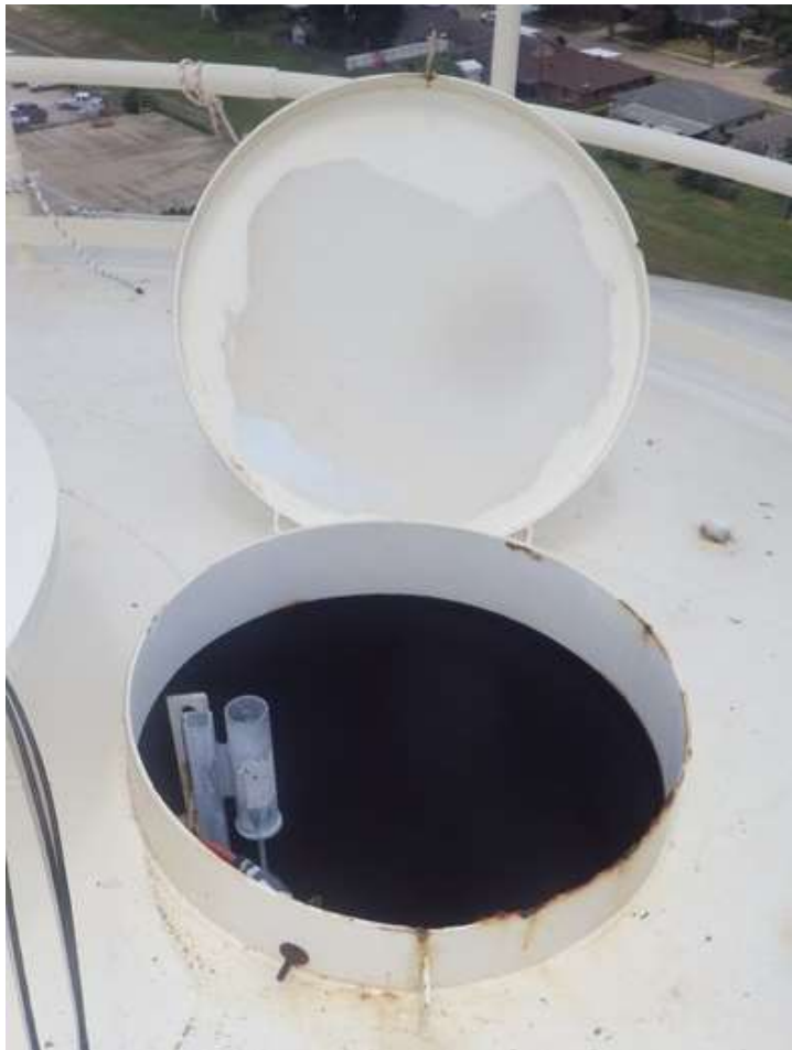
41. Misaligned container roof manhole locking hasps.
