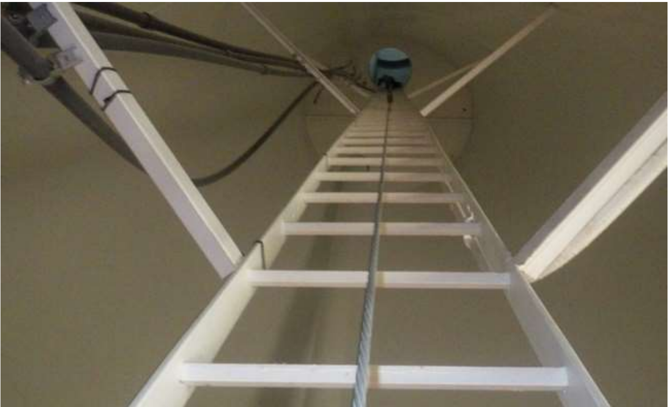
62. Base cone ladder, safe-climbing device, and brackets.
