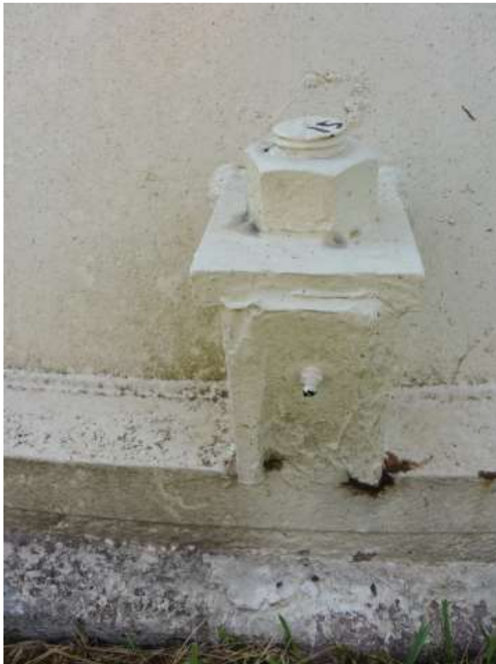
9. Buried foundation, grout, base plate, and anchor bolt chair.
