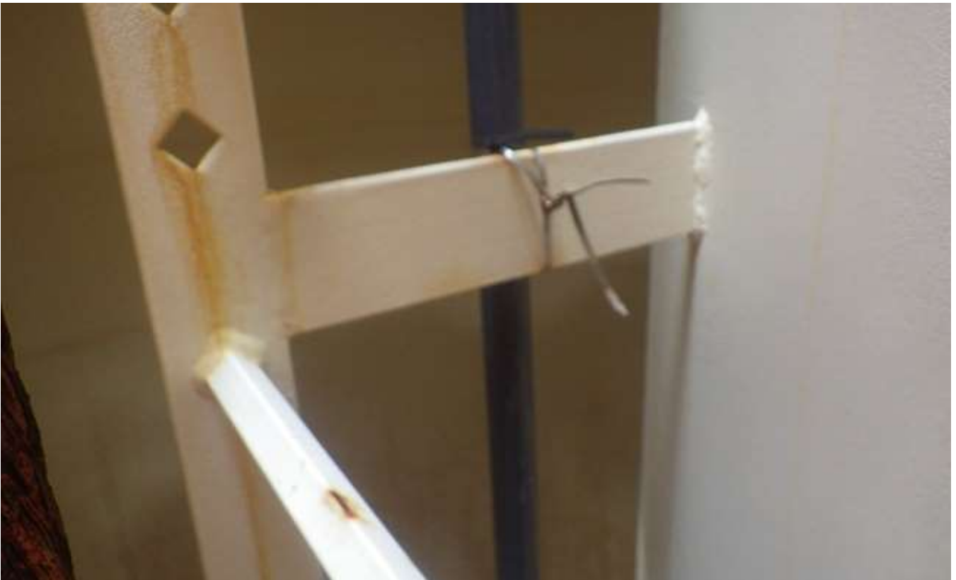
100. Conduit attached to the interior wet container ladder bracket.
