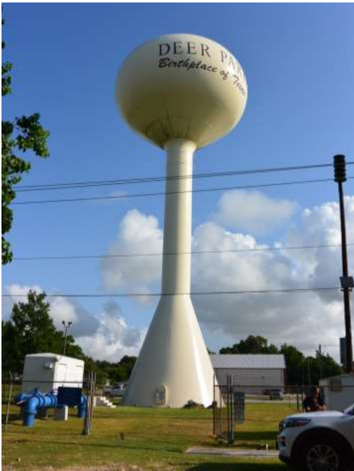
2. Tank and site.
