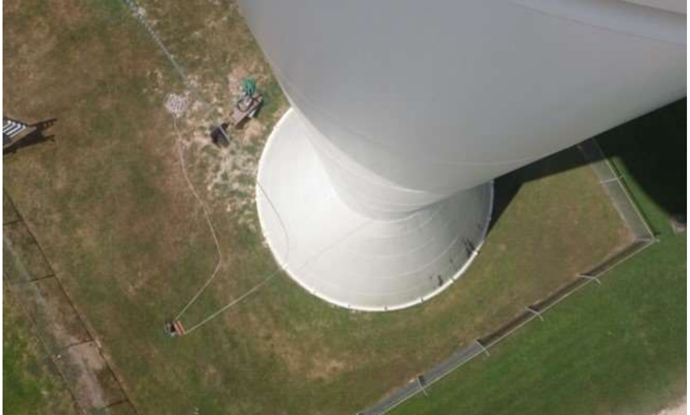
16. Base cone and support column exterior.
