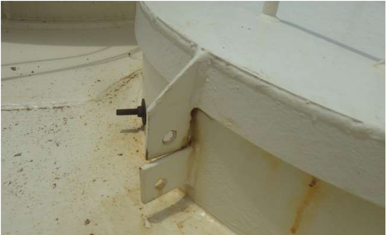
41. Misaligned container roof manhole locking hasps.
