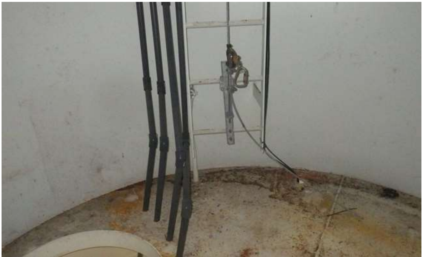
68. Support column ladder, safe-climbing device, and cables.
