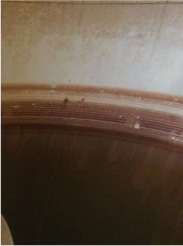
103. Water and silt on the interior wet bowl.
