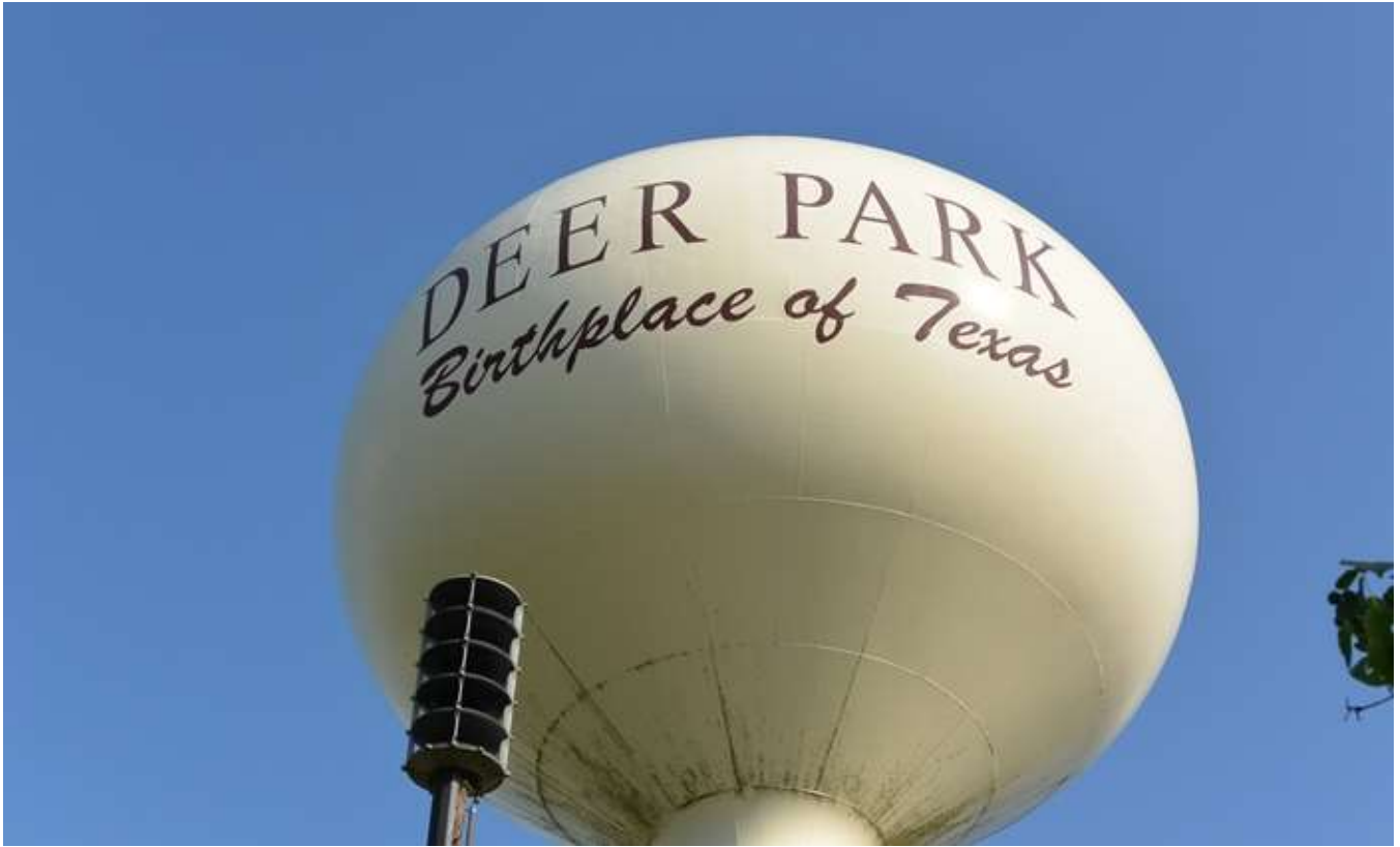
25. Mildew on the bowl exterior and signs on the shell exterior.
