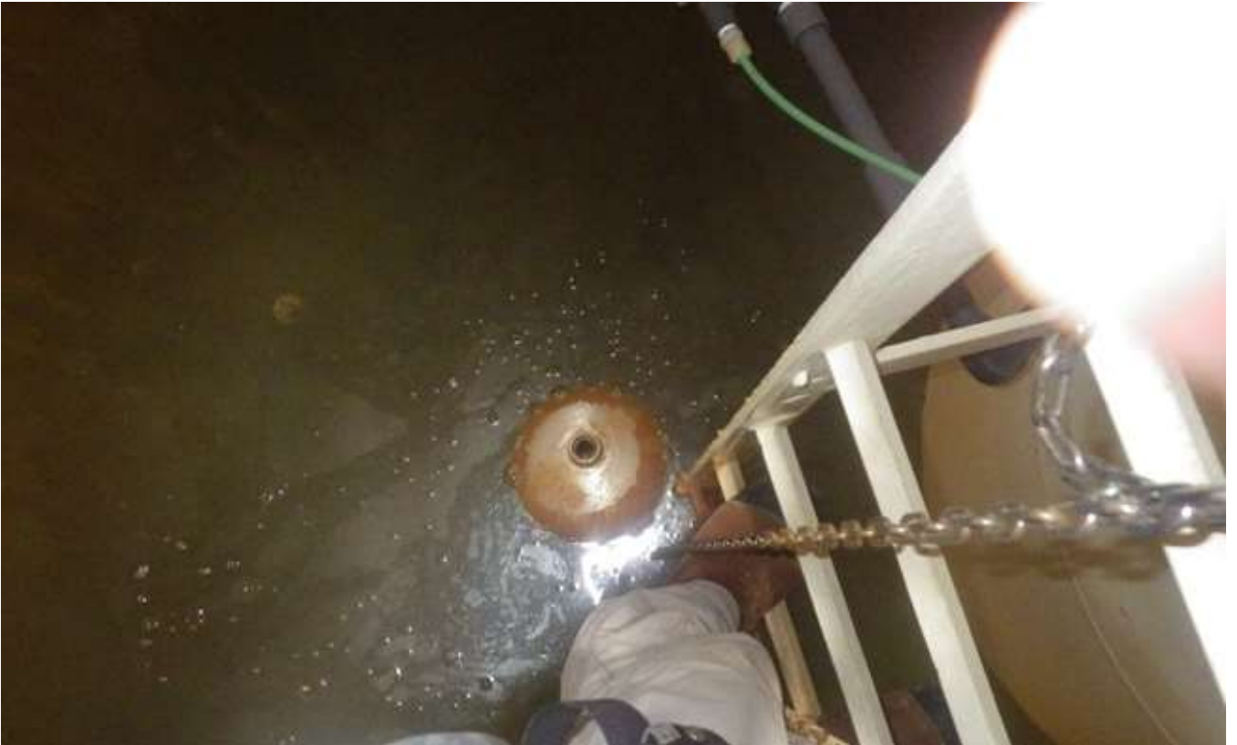
102. Equipment suspended inside the container.
