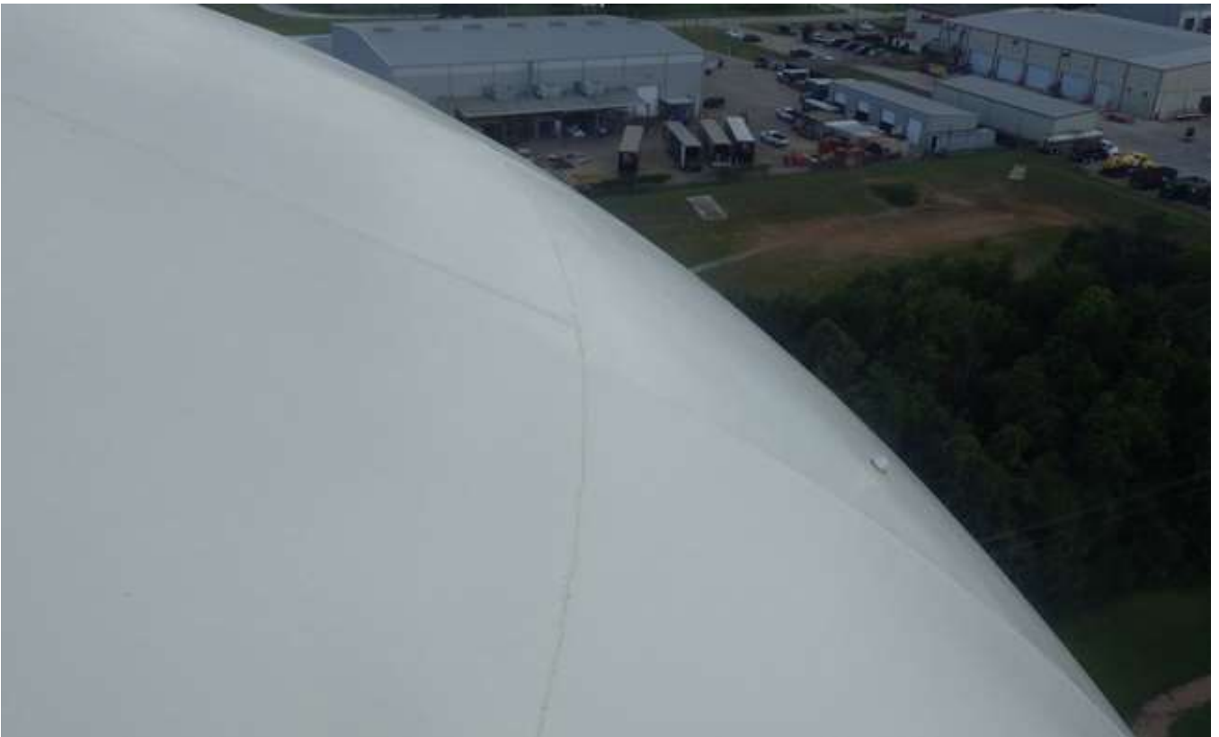
28. Threaded and plugged coupling in the roof exterior.
