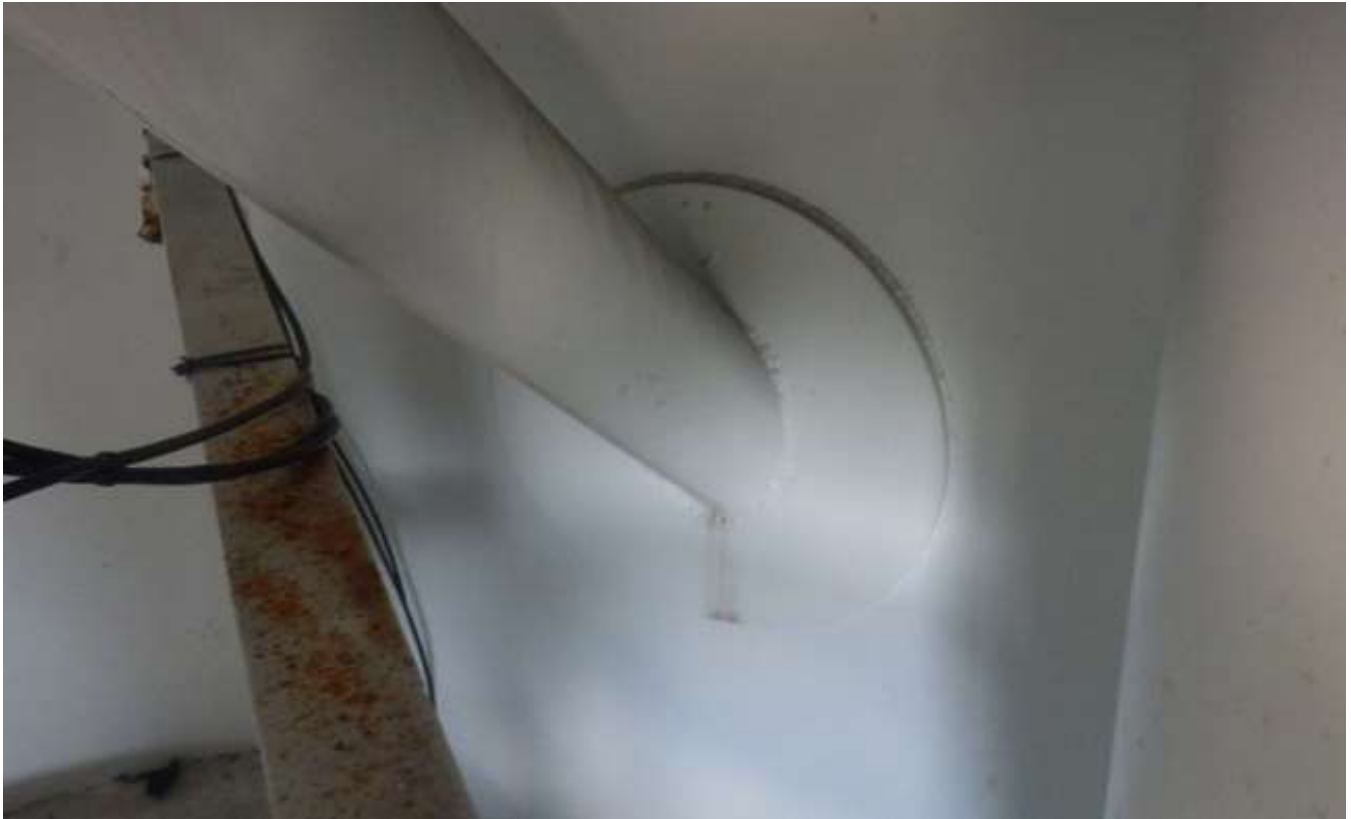
72. Overflow pipe penetrating near the top of the support column.
