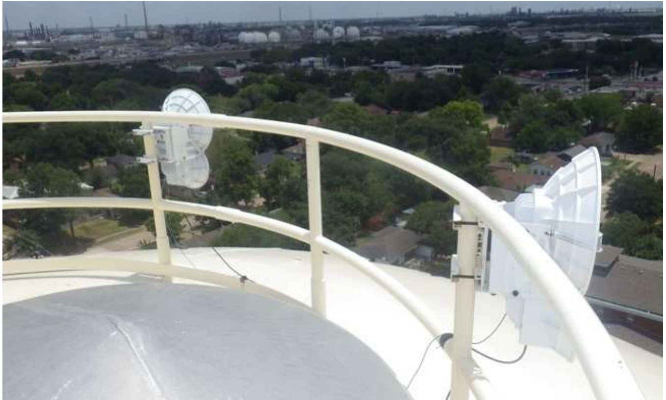
34. Antennas attached to the roof safety railing.
