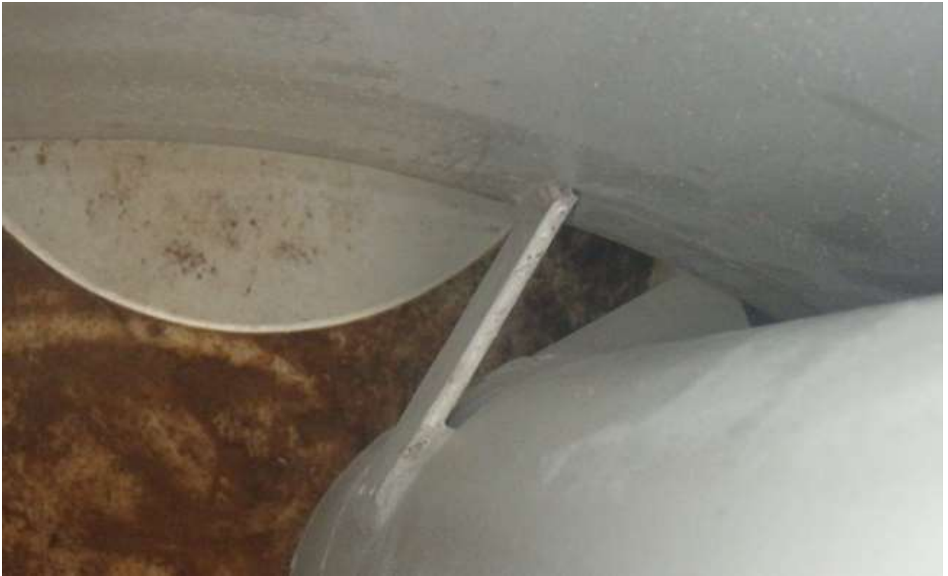
73. Overflow pipe bracket welded to the interior dry access tube.
