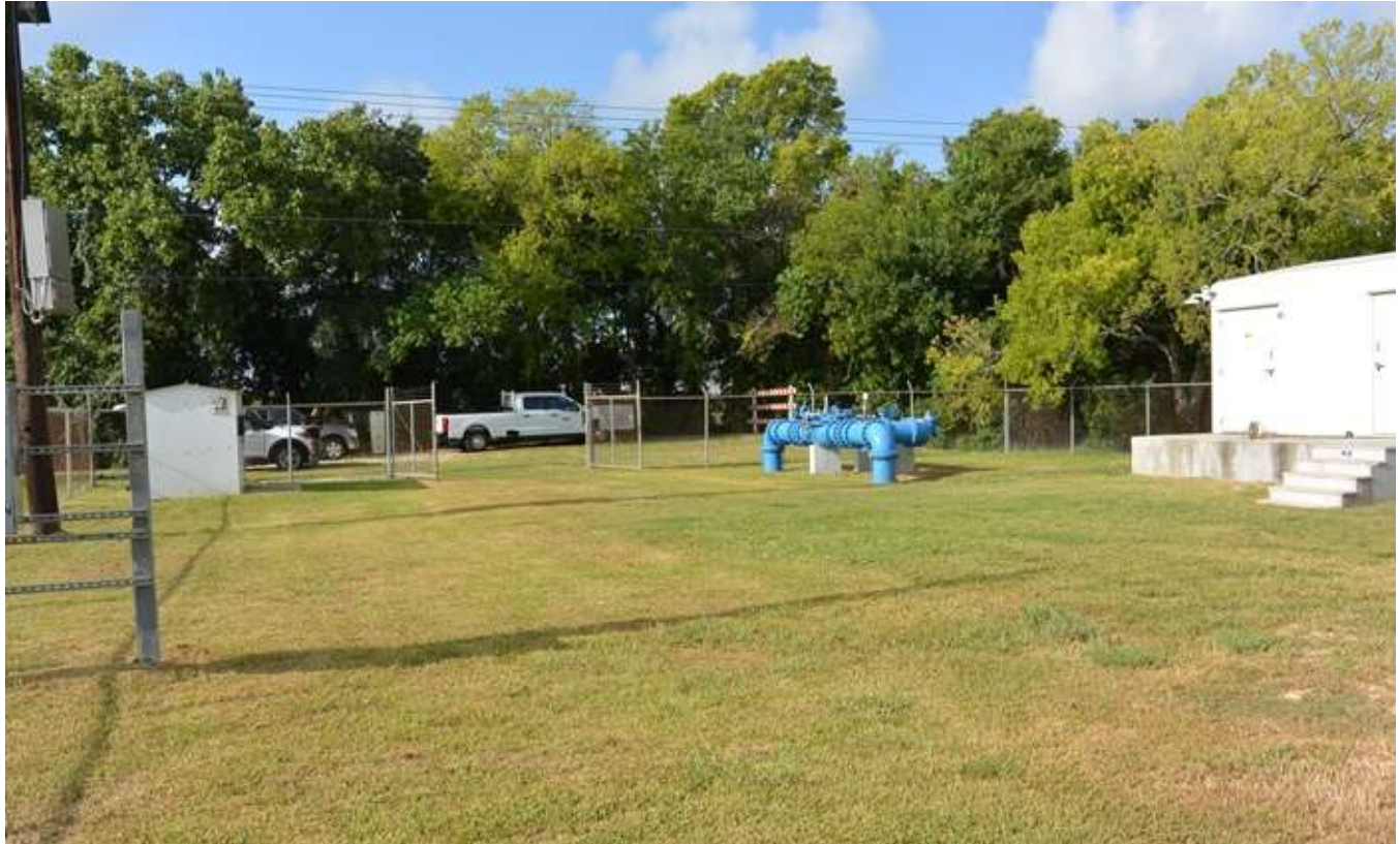
6. Piping and building on site.
