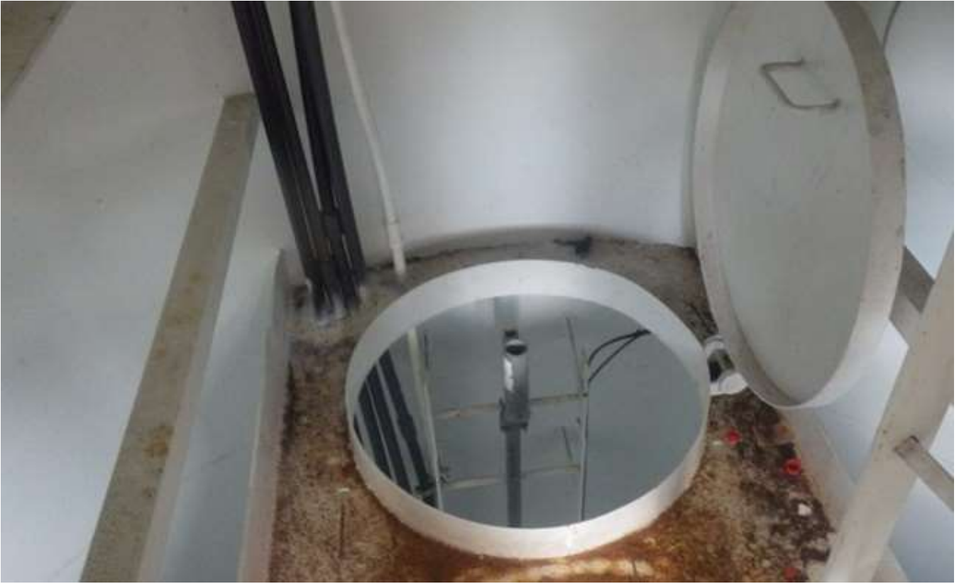
71. Top platform manhole.
