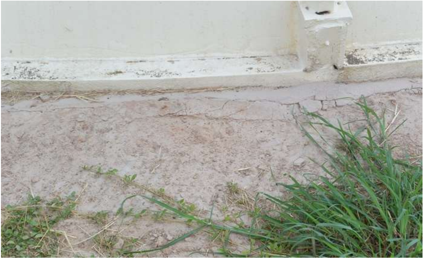
9. Buried foundation, grout, base plate, and anchor bolt chair.
