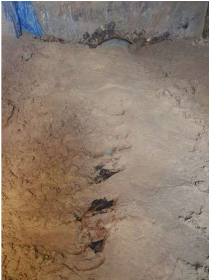
49. Exposed piping at the severely damaged base cone floor.
