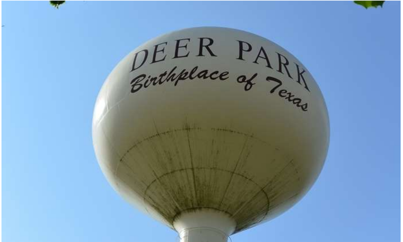
24. Mildew on the bowl exterior and signs on the shell exterior.
