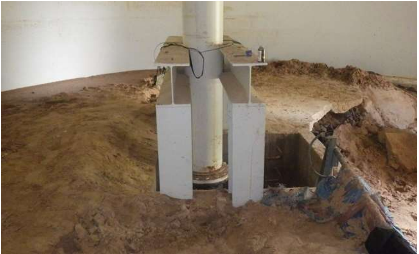
55. Inlet/outlet pipe extending from pipe pit in the base cone floor.
