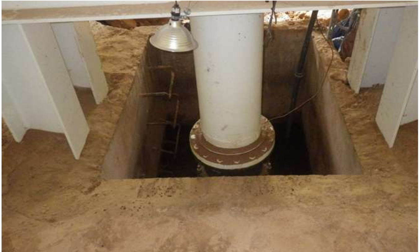
58. Inlet/outlet pipe extending from the pipe pit.
