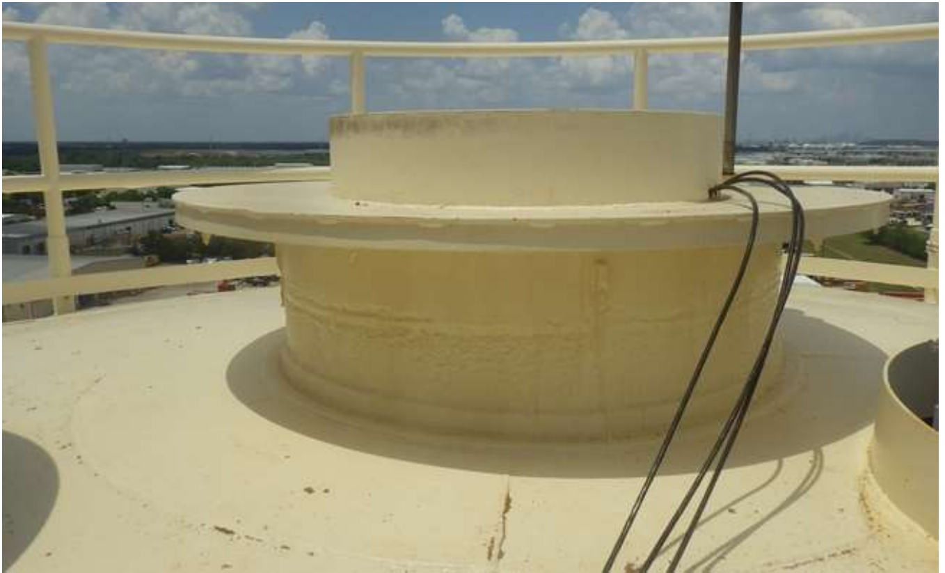
37. Access tube roof manhole. Note cables extending through the manhole curb.
