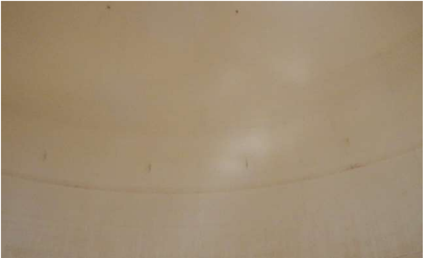
89. Roof and shell interior.
