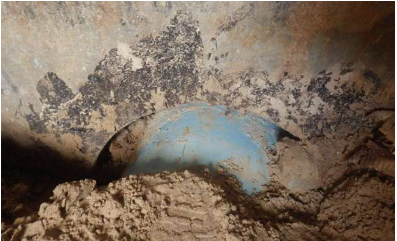
49. Exposed piping at the severely damaged base cone floor.
