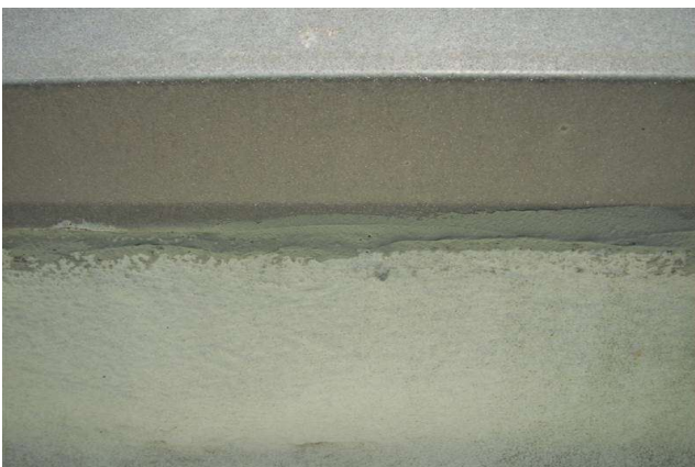
Sealed wall joint.
