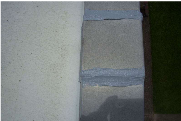
Sealed wall joints.
