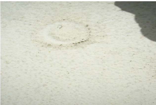
Fastener backout.
