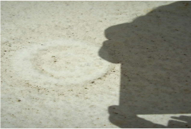
Fastener backout.
