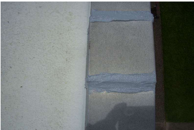
Sealed wall joints.
