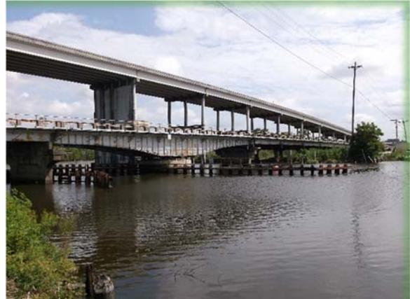
Gibson & Associates, Inc. was contracted by the Texas Department of Transportation to repair and refurbish the SH 73 over Cow Bayou Swing Bridge in Orange, Texas. This bridge is a steel I Beam bridge that was built in 1938 to allow both vehicular and large marine traffic to navigate the bayou. Due to the lack of large marine traffic and advanced age of the bridge, the mechanical equipment in the swing portion of the bridge was allowed to fall into disrepair.
