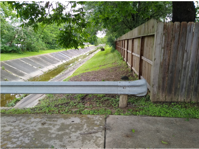
The existing guardrail at the intersection of the drainage easement and East P Street will need to be modified in order to provide access for the proposed trail.
