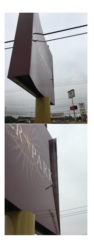
Example 1: Sign shows a significant bend in the back panel. Bolts protruding out the back side.
