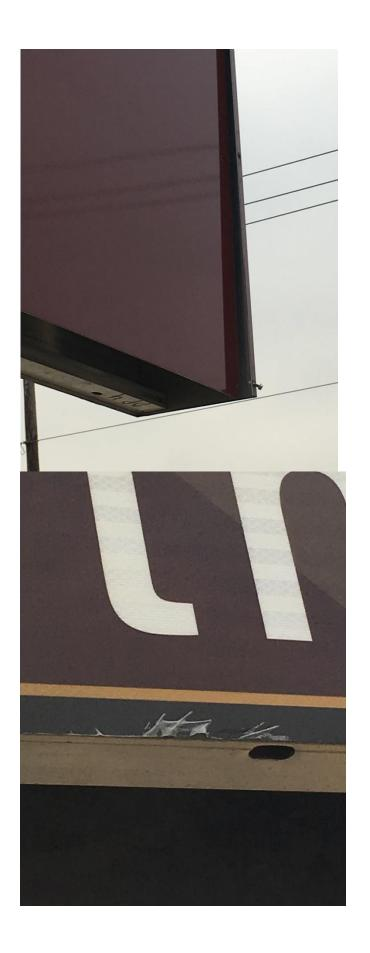
Example 7: Back panel is separating from the existing frame. Rivets popping out.
