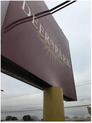
Example 4: Sign shows significant bend in back panel.
