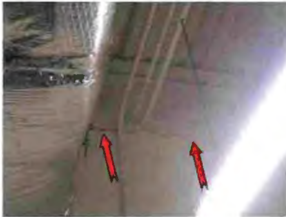
Photo #73 Crack in gypsum wallboard wall
