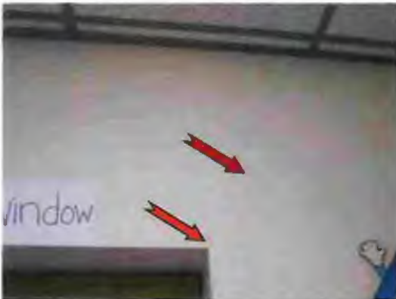
Photo #57 Crack in gypsum wallboard wall
