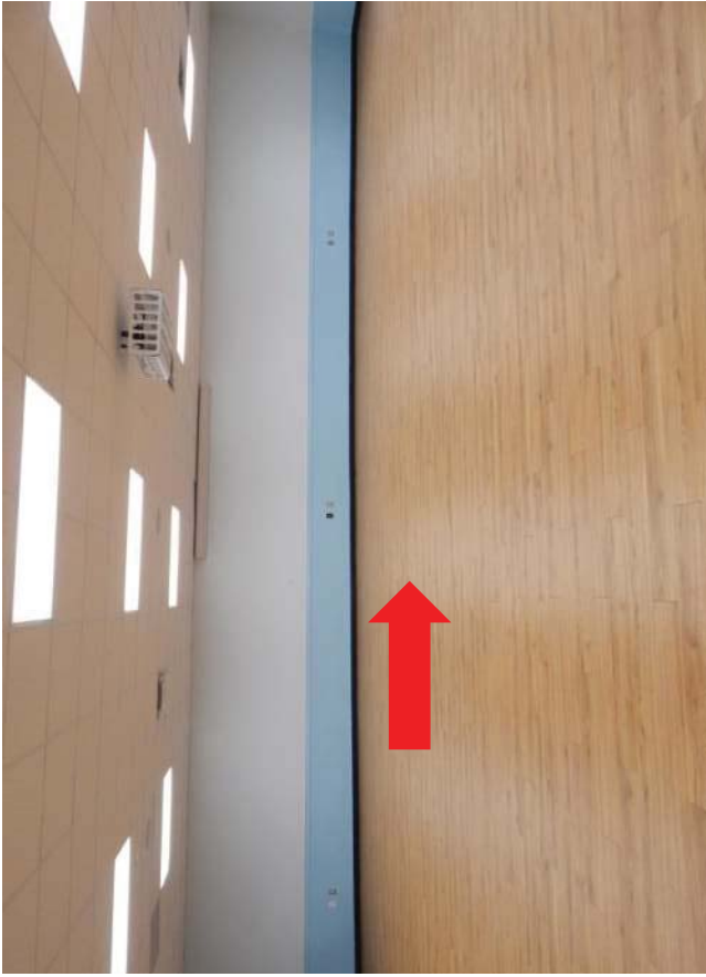
#42 A visible hump up of the floor can be seen in this area
