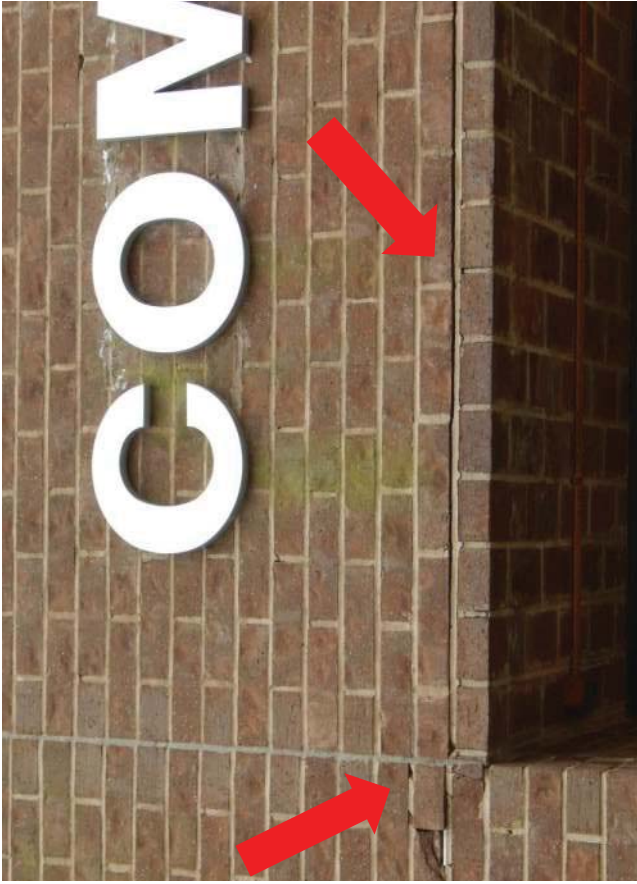
#13 Horizontal crack between brick soffit and brick on face of building. Cracking brick where lintel angle is bearing on brick column.
