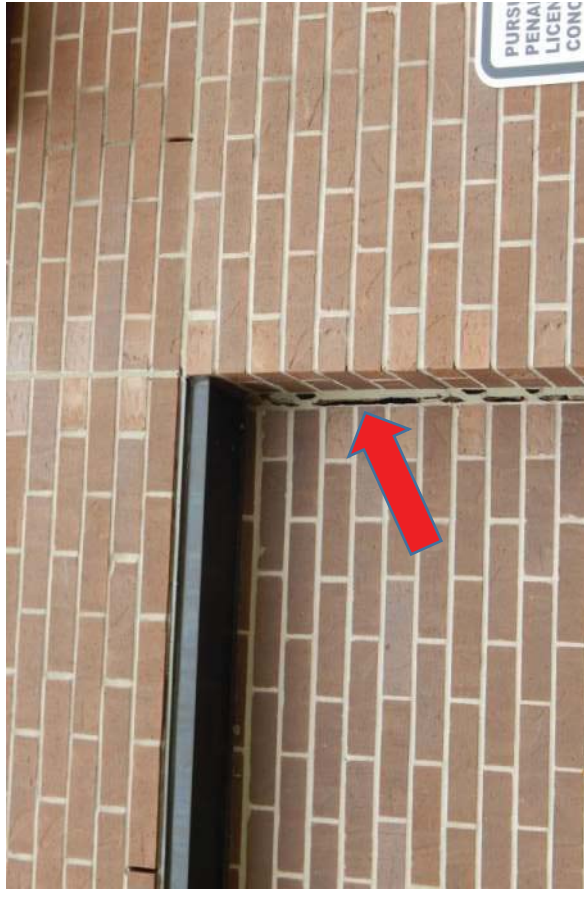
#24 Separation in caulk joint at end of inset brick panel of approximately 1/2". No separation in control joint above.
