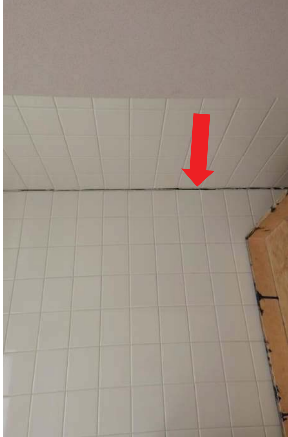
#37 Cracking and separation in tile
