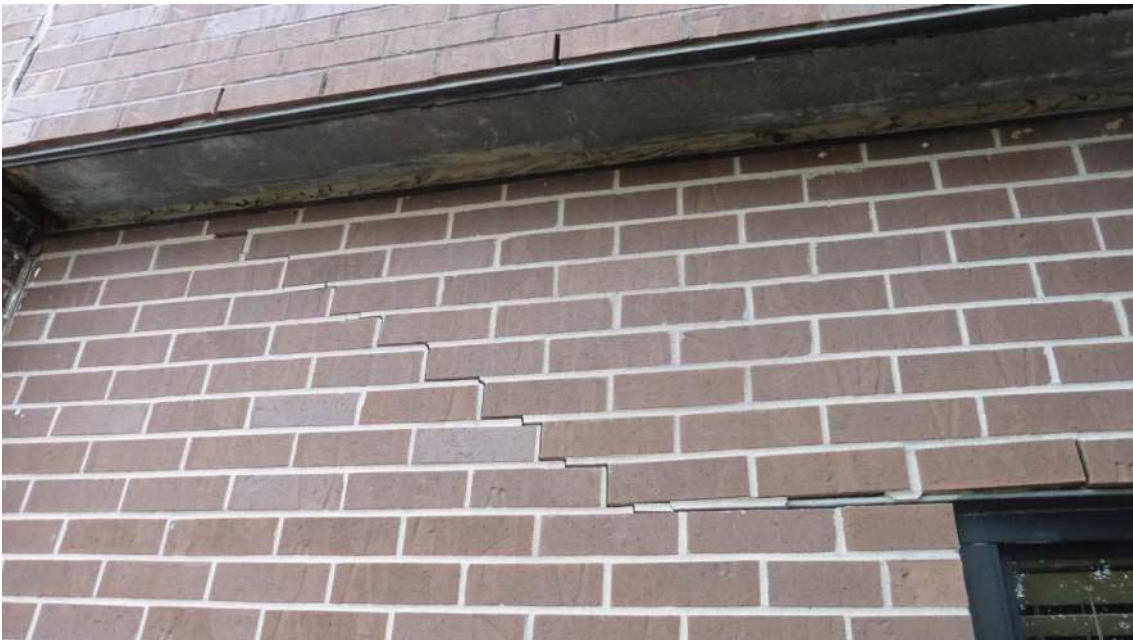
Examples of structural movement damage
