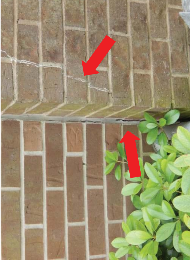
#10 Same as photo #9 at bottom of crack repair and separation in caulk joint.
