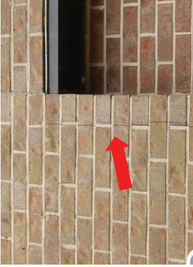
#14 Vertical crack where steel lintel over inset brick is Moving and dragging the brick on the column
