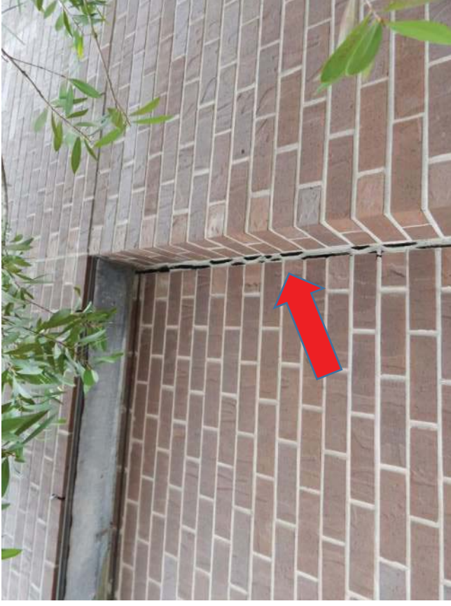
#18 Separation in caulk joint at end of inset panel. Crack does not go up in control joint above inset panel. Separation at top was measured at approximately \frac{1}{2} "
