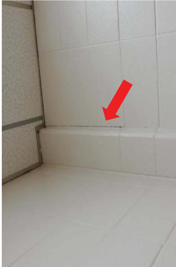
#44 Crack in corner of CMU wall
