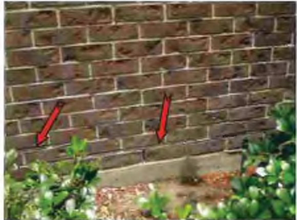
Photo #22 Masonry-mortar-joint crack
