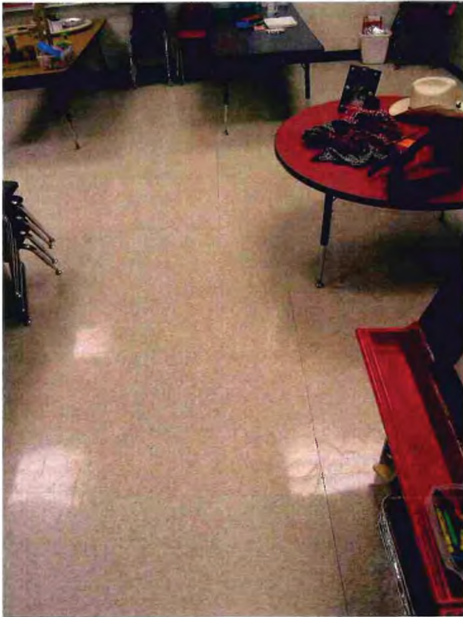
Photo 2. Separation of floor tiles in addition.
