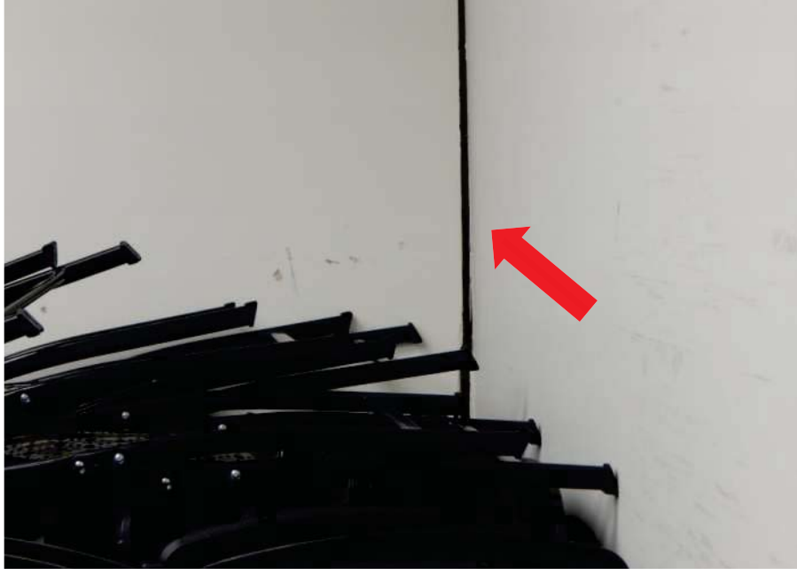
#33 Separation of base of wall to floor
