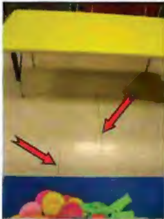
Photo #61 Separations in vinyl tile floor
