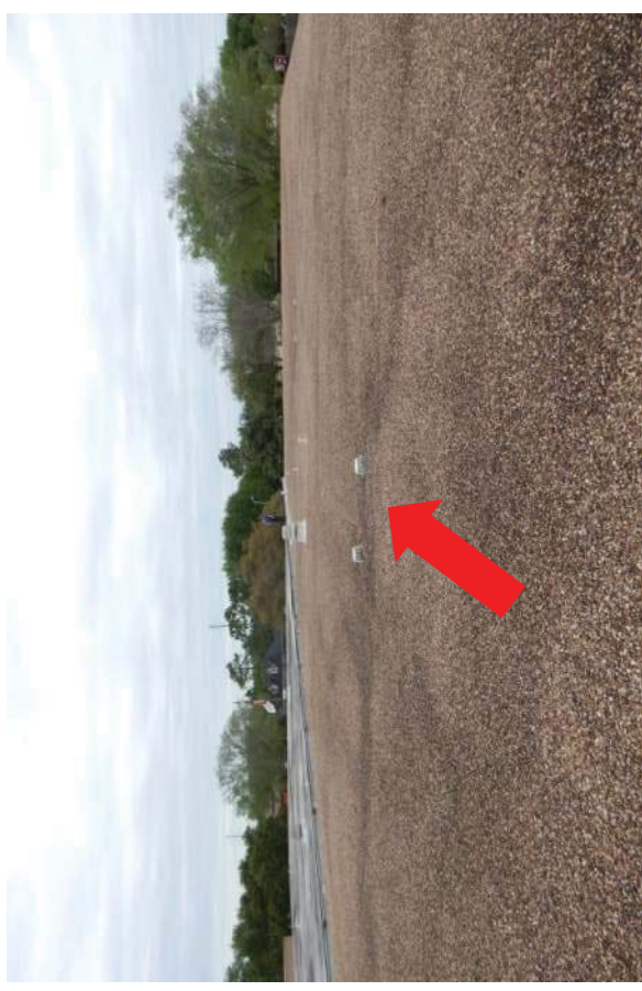
#53 Roof over phase two of community center showing roof drain and emergency drain
