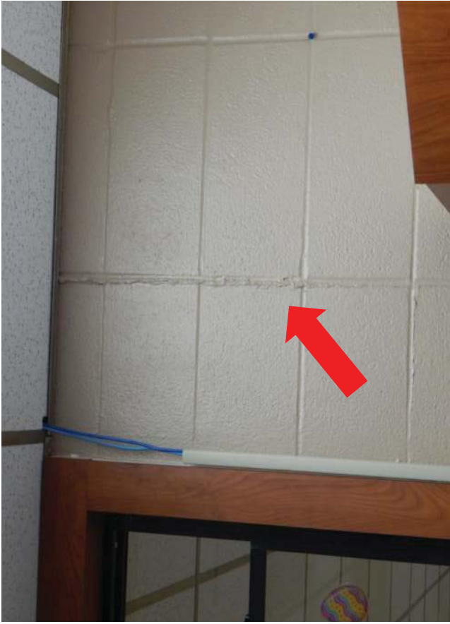
#50 Vertical crack in CMU wall
