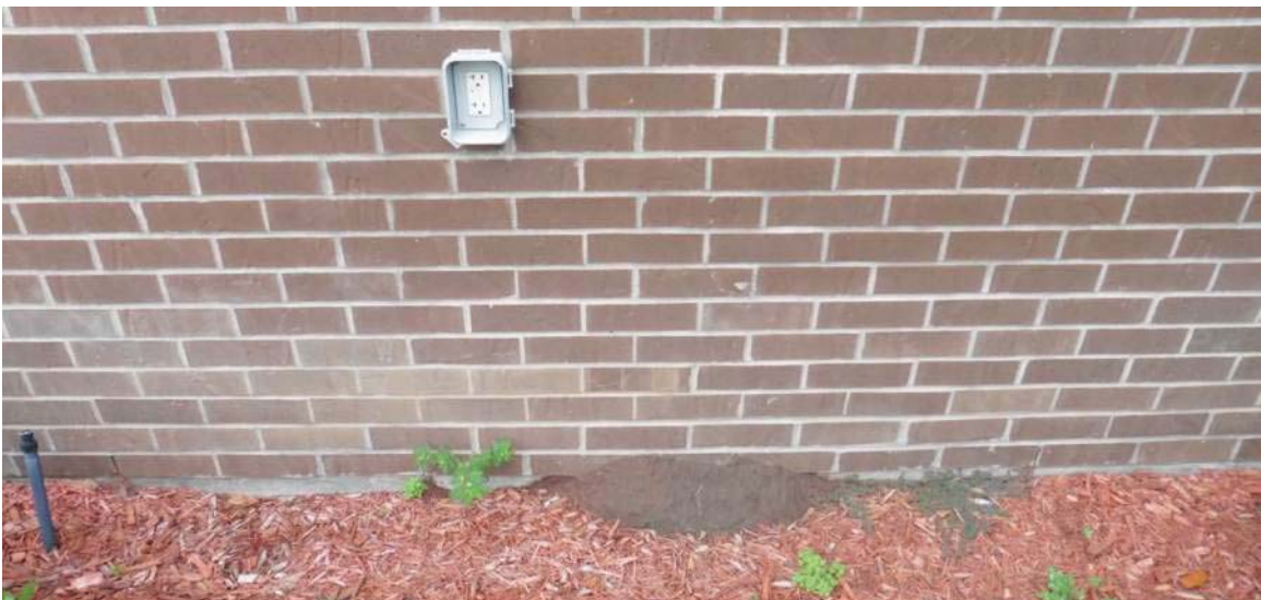
Insect infestation, and example of unprotected electrical
