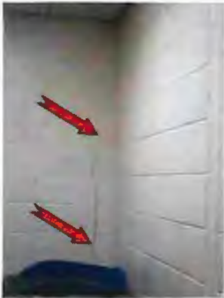
Photo #25 Crack through concrete masonry unit wall
