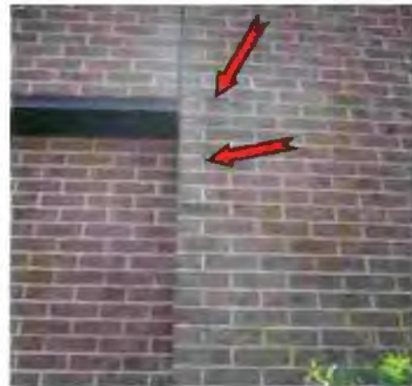
Photo #8 Masonry-mortar-joint crack
