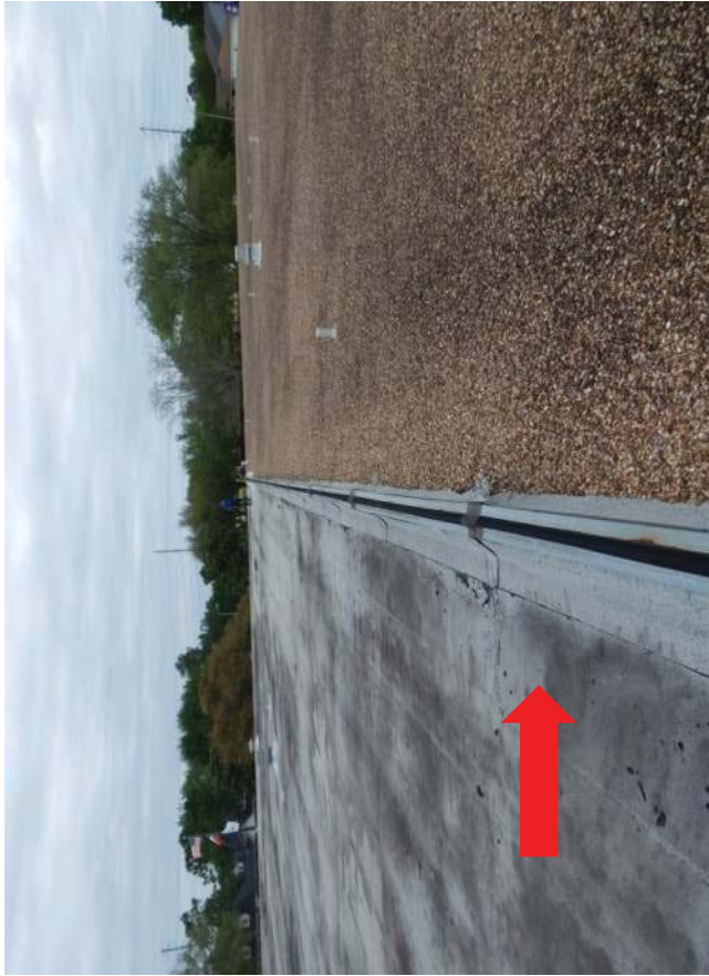
#54 Roof expansion joint cover between phase one and phase two
