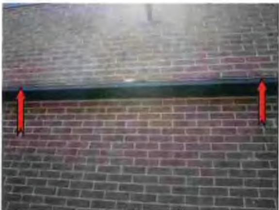
Photo #5 Separation between the brick veneer and the metal flashing
