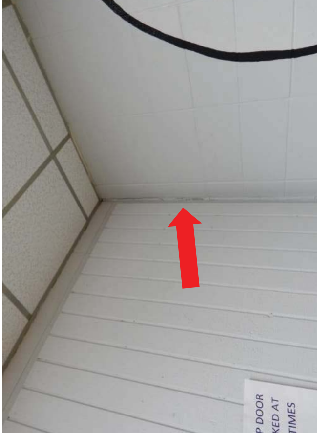
#47 Crack in corner of CMU wall
