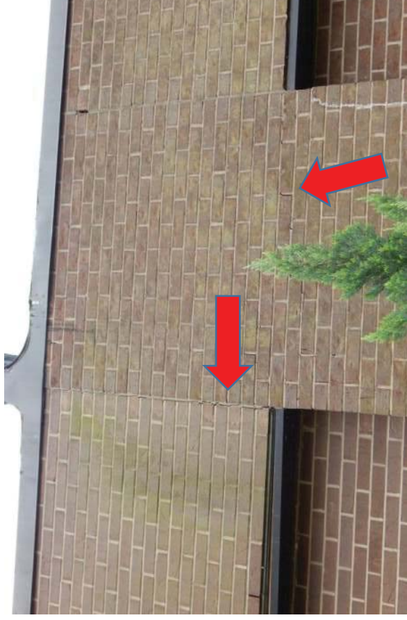
#8 Control joint between phase one (on right) and phase two (on left) showing separation in joint. Also, there is a step crack in the brick.
