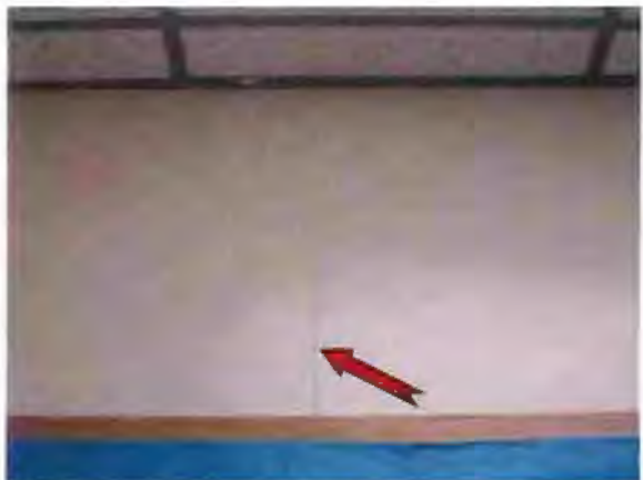
Photo #72 Crack in gypsum wallboard wall
