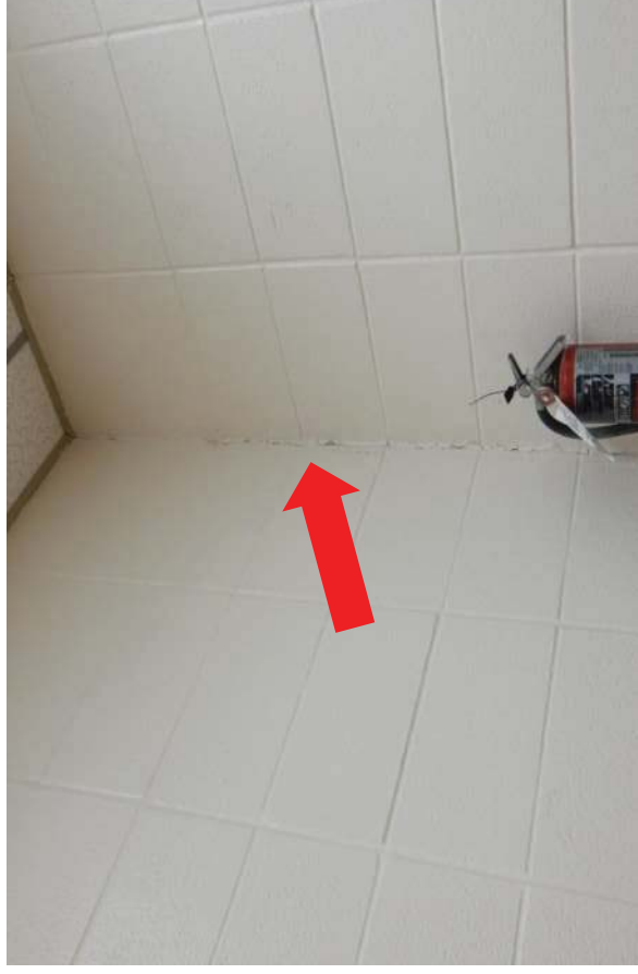
#43 Level on floor showing sloping down toward the North East corner at Approximately 1/8" per foot
