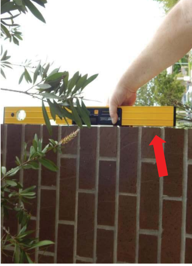
#22 Showing how brick column is leaning outward at the top of the East
