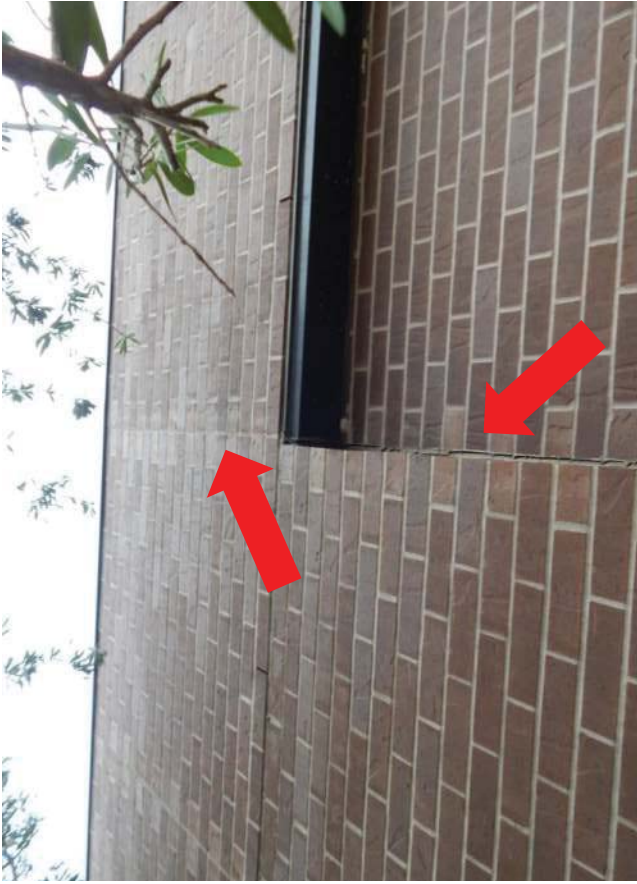
#17 Separation in caulk joint at end of inset panel. Crack does not go up in control joint above inset panel
