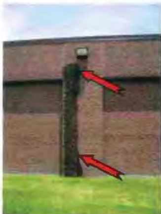
Photo #23 Staining on exterior brick veneer
