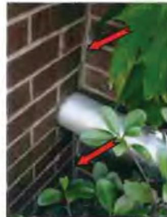
Photo #10 Separation at expansion joint
