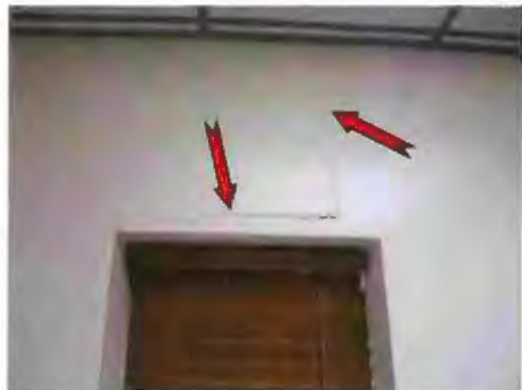
Photo #66 Crack in gypsum wallboard wall
