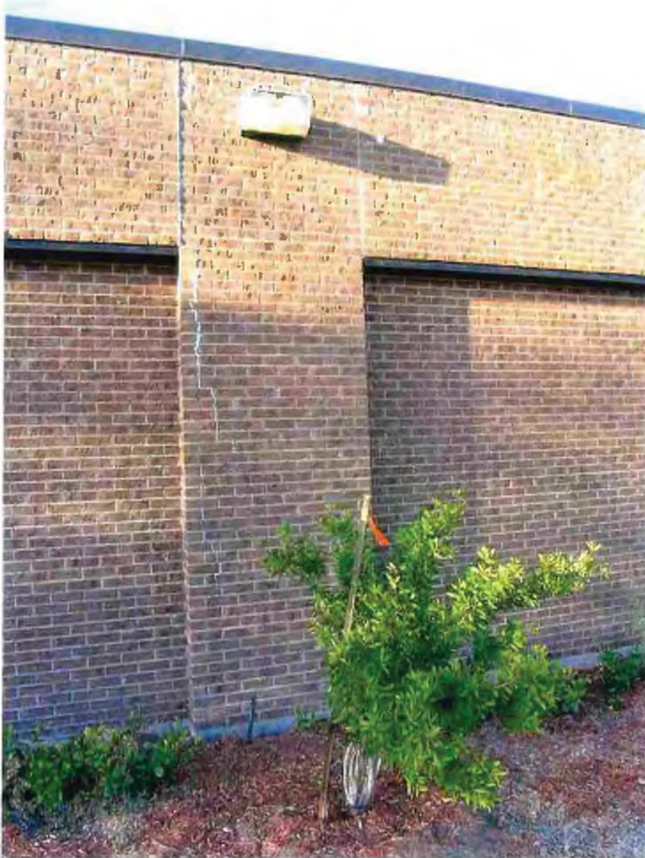
Photo 5. Exterior façade cracks (in original building) closing at top.
