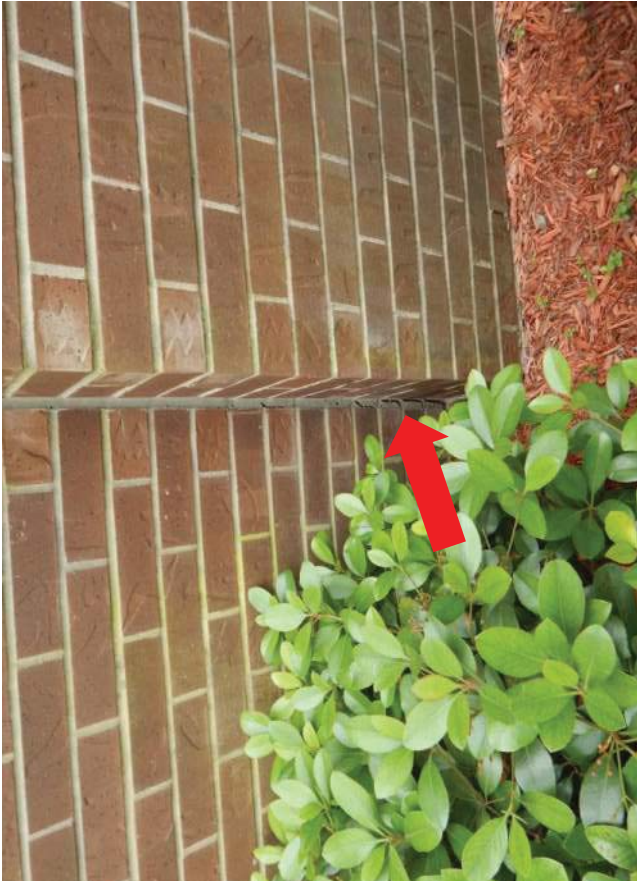
#5 Minor separation in caulk joint at end of inset panel.
