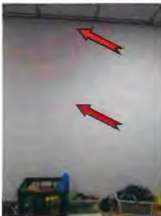
Photo #59 Crack in gypsum wallboard wall
