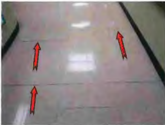
Photo #45 Separations in vinyl tile floor
