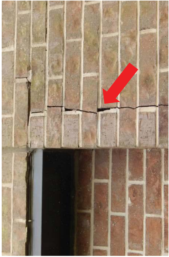
#12 Same location as photo #11 showing cracked brick in column. Lintel movement is causing this cracking.
