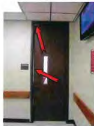
Photo #42 Door out-of-square with respect to its frame and binding in its frame
