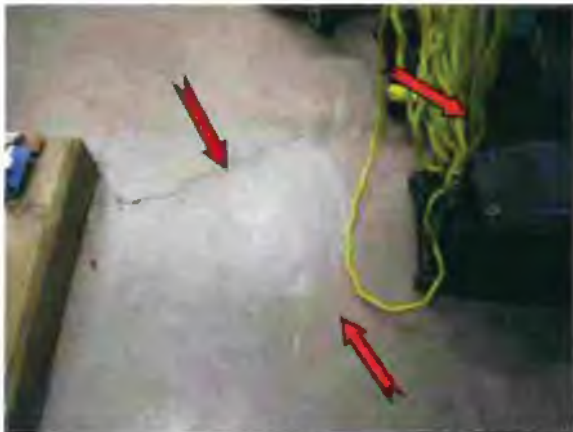
Photo #75 Cracks in exposed concrete floor
