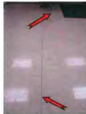
Photo #60 Separations in vinyl tile floor
