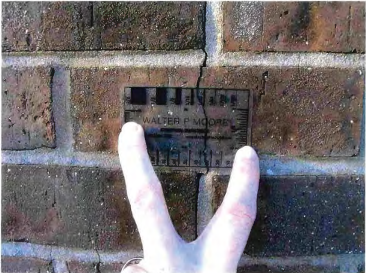
Photo 3. Exterior façade crack (in original building) near grade.
