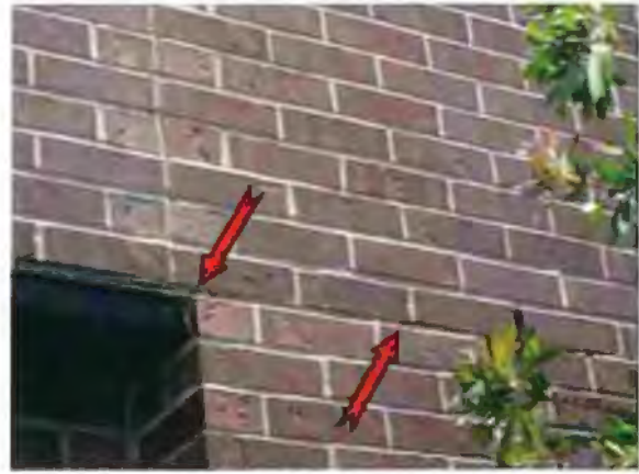
Photo #16 Separation at expansion joint
