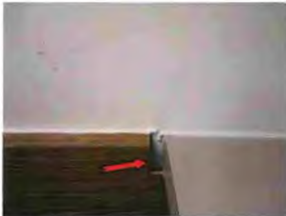
Photo #63 Separation between wood trim and counter top
