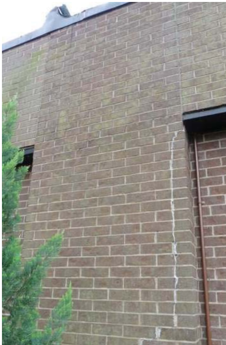
Examples of movement damage
