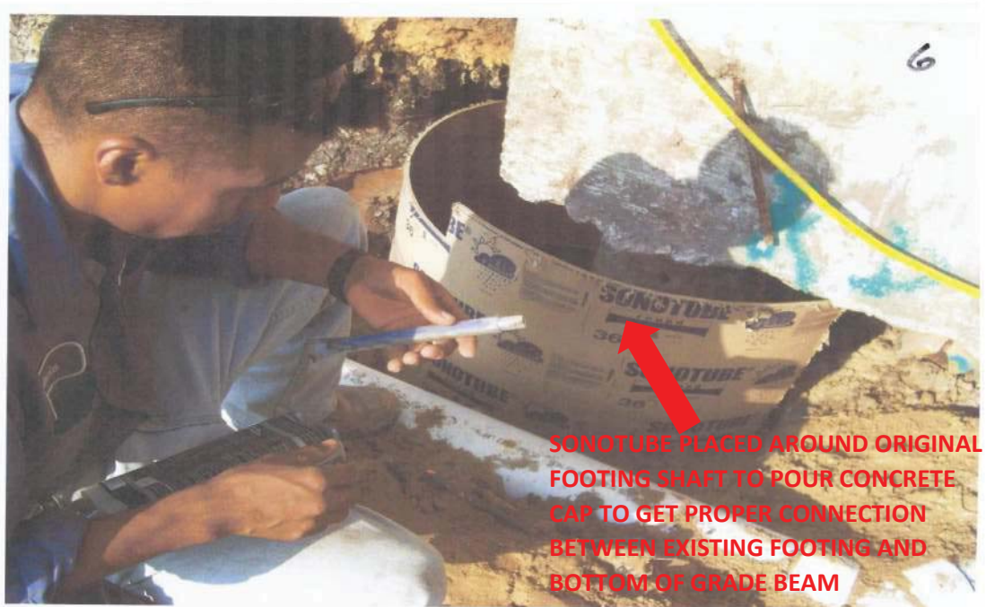
#5 Photo taken by contractor of Phase Two showing how concrete cap was being poured between existing footing and grade beam
