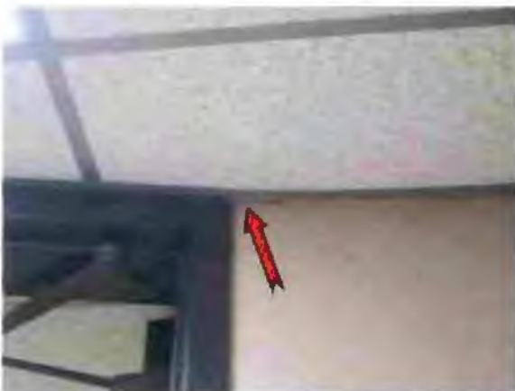
Photo #41 Separation between the gypsum wallboard and the suspended acoustical ceiling
