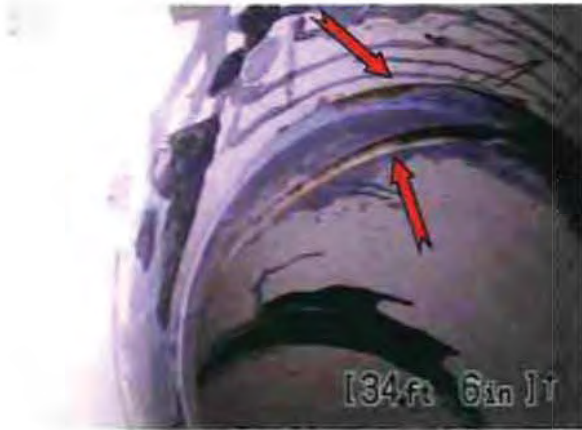
Photo #79 Broken pipe a in the 12-inch PVC storm line for the original building
