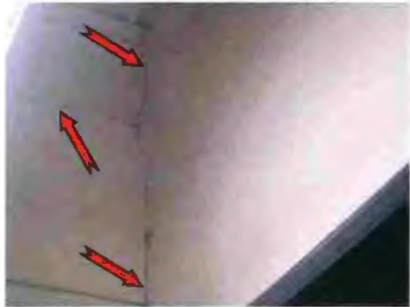
Photo #74 Crack in gypsum wallboard wall
