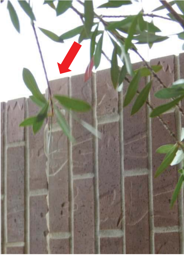
#21 Showing brick column has moved outward to the East approximately 1"
