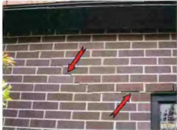
Photo #20 Masonry-mortar-joint crack
