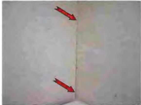
Photo #56 Crack in gypsum wallboard wall
