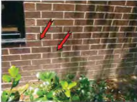
Photo #19 Masonry-mortar-joint crack
