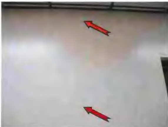
Photo #65 Crack in gypsum wallboard wall
