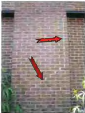
Photo #9 Masonry-mortar-joint crack
