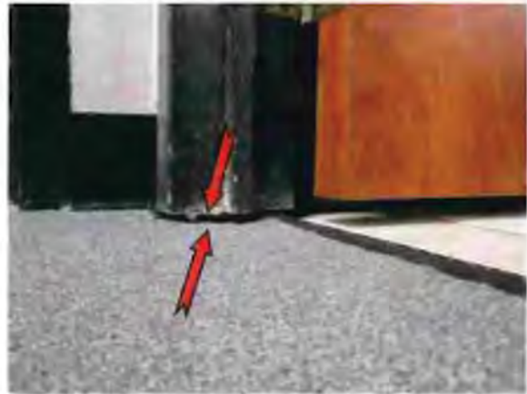
Photo #26 Separation between door frame and floor
