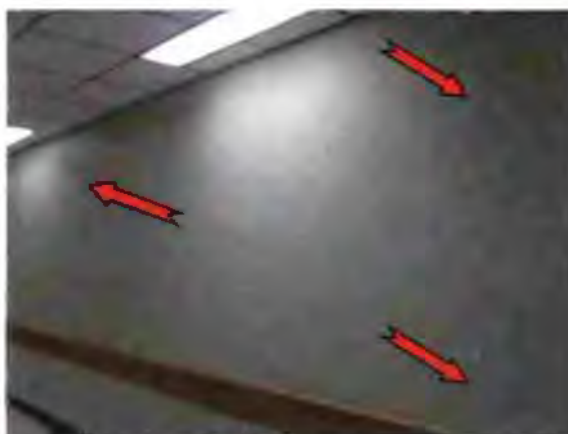
Photo #32 Cracks in gypsum wallboard wall
