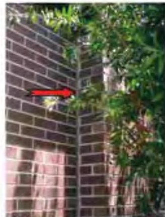
Photo #18 Separation at expansion joint
