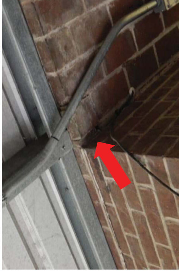
#16 Crack in brick of soffit brick same as photo #13
