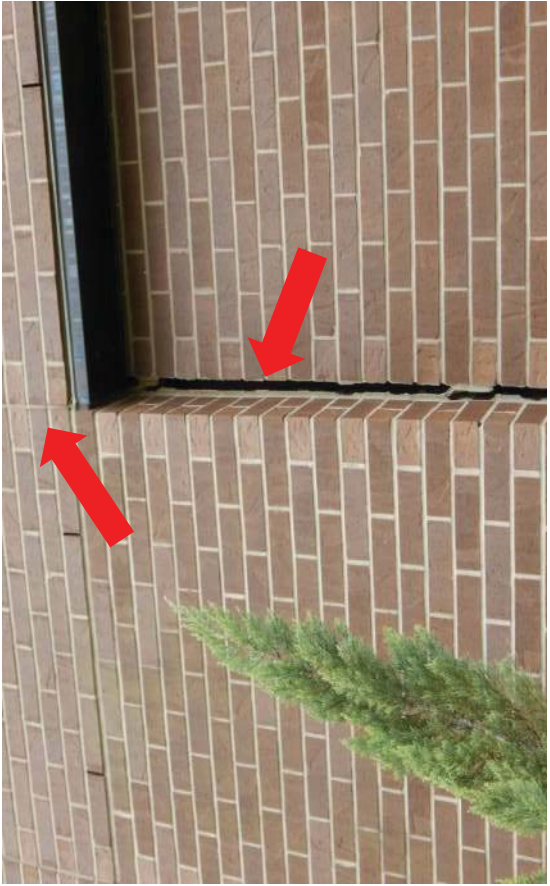
#3 Separation in caulk joint at end of inset brick panel of approximately 1". No separation in brick control joint above.
