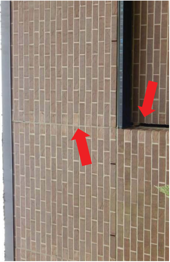
#4 Separation in caulk joint at end of inset brick panel of approximately 1". No separation in brick control joint above.
