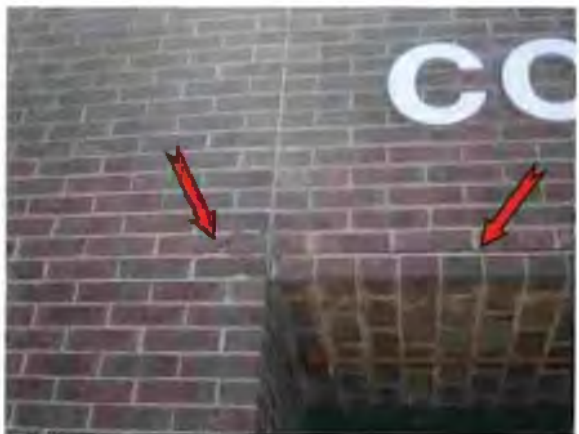
Photo #6 Masonry-mortar joint crack
