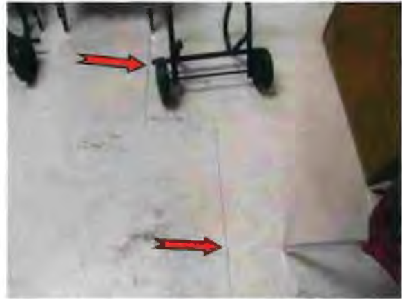
Photo #50 Separations in vinyl tile floor
