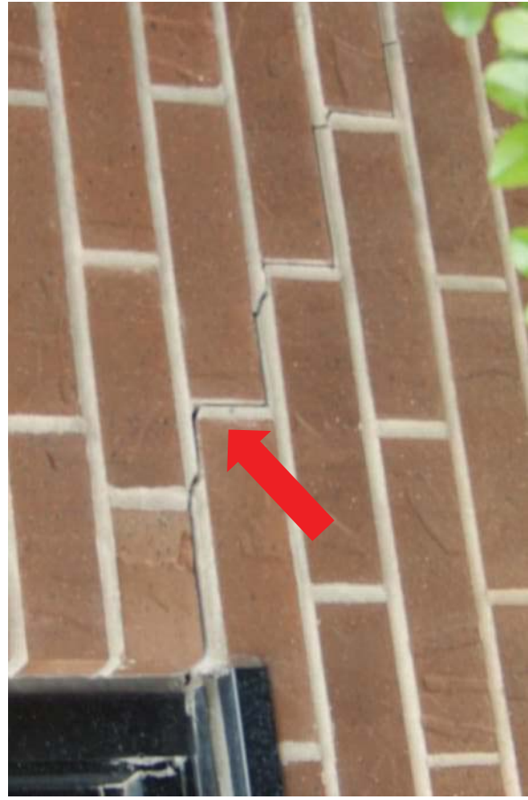
#26 Photo at connection of phase one and phase two buildings. Separation of caulk joint between phase one and phase two. Brick cracking and being pushed out on phase one building.
