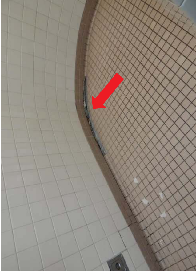
#34 Cracking in the tile floor at base of wall
