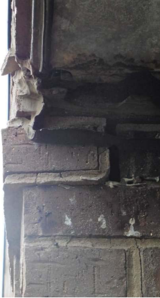
Examples of movement damage
