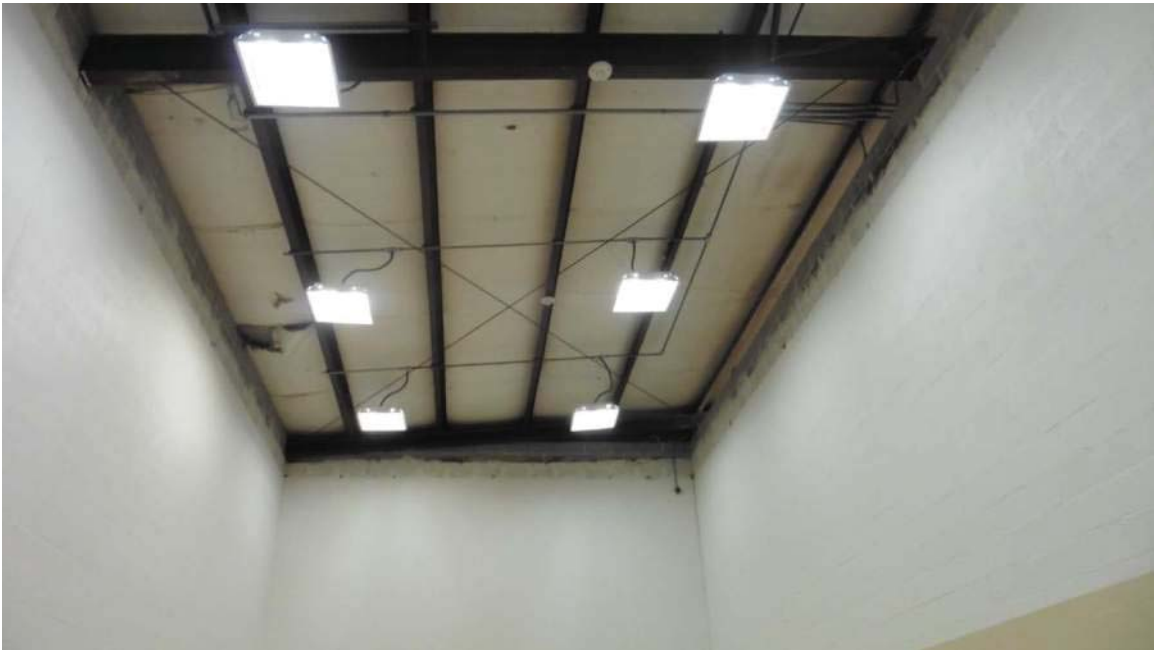
Examples of damaged “over-the-purlin” gym roof insulation
