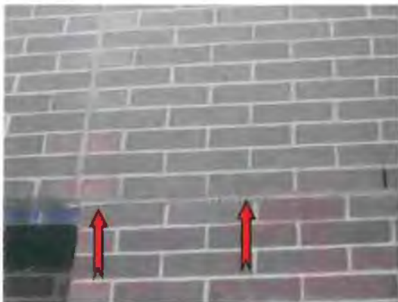
Photo #11 Separation at expansion joint
