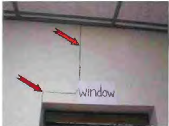
Photo #58 Crack in gypsum wallboard wall
