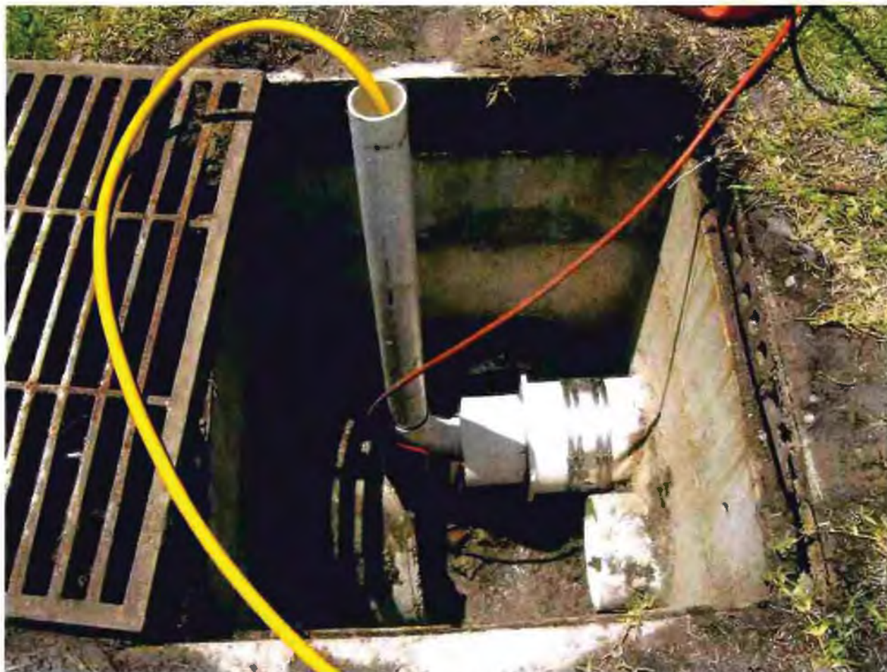
Photo 7. Leak testing of underground 10-inch diameter main roof drain for addition.
