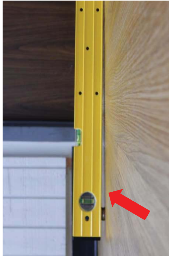
#49 Level on floor showing a slope of approximately 3/16 inch per foot
