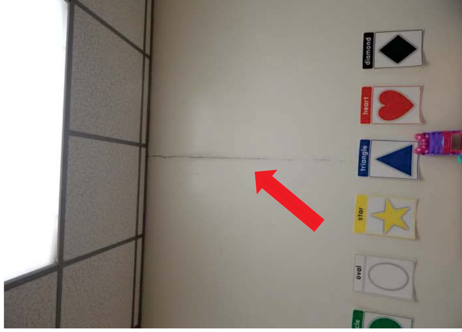
#38 Cracking in sheetrock
