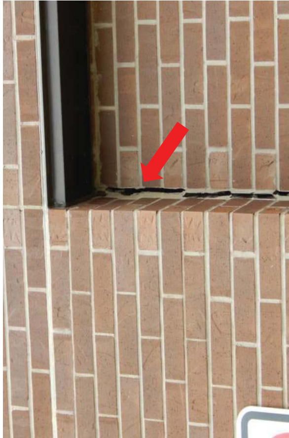
#23 Separation in caulk joint at end of inset brick panel of approximately 1/2". No separation in control joint above.
