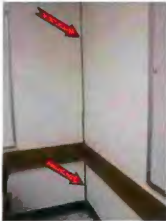
Photo #49 Separation in gypsum wallboard wall
