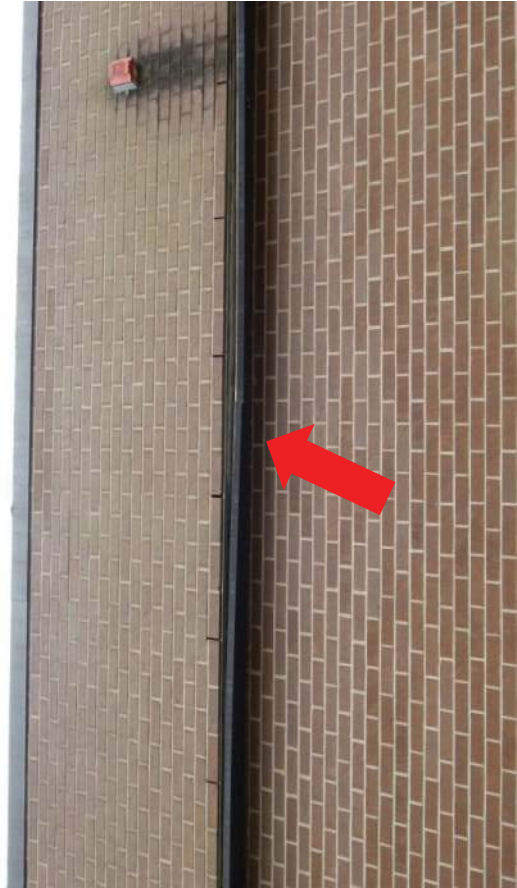
#7 Sheet metal soffit is sagging down. This is where the brick header was omitted and sheet metal added (typical).
