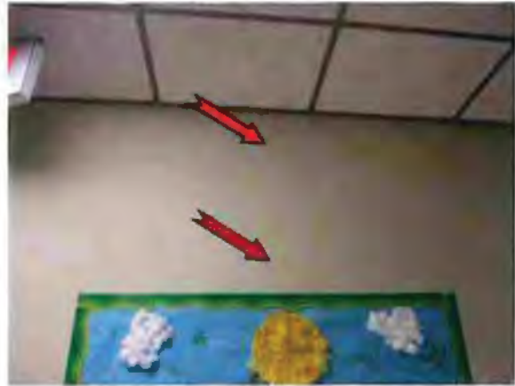
Photo #44 Crack in gypsum wallboard wall
