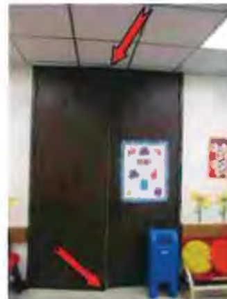
Photo #54 Door out-of-square with respect to its frame and binding in its frame
