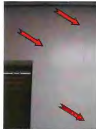
Photo #64 Cracks in gypsum wallboard wall
