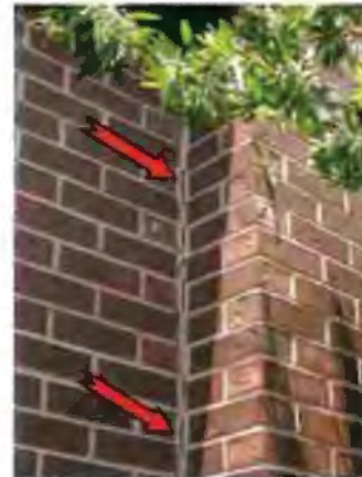
Photo #14 Separation at expansion joint
