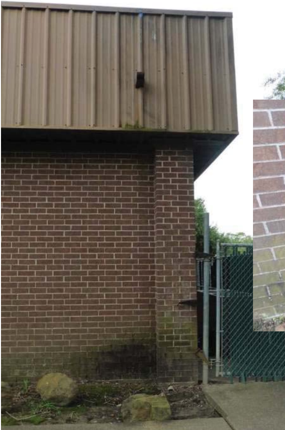
Mildew growth and damaged electrical
