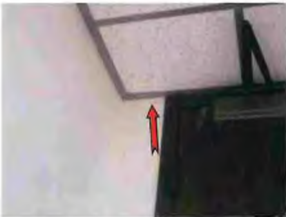
Photo #47 Crack in gypsum wallboard wall
