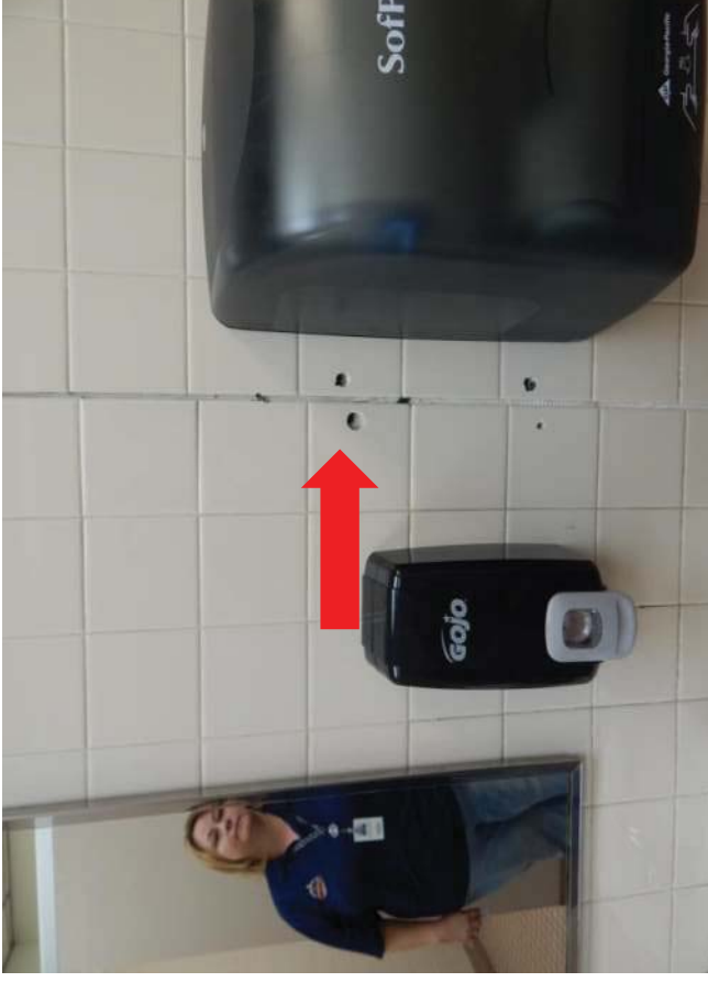
#36 Cracking and movement in tile joint. Mrs. Crenshaw said towel dispenser had to be moved.
