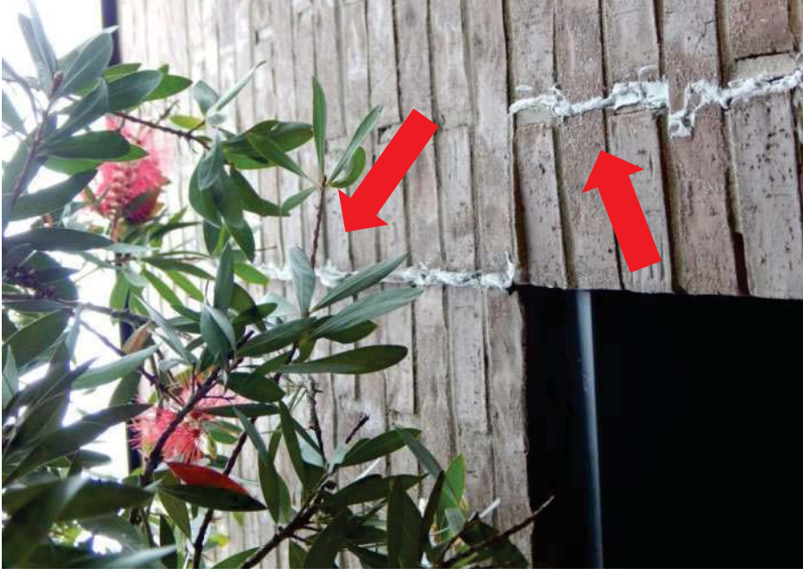
#30 Photo at same location as photo #29 at the corner of the inset brick Panel. Repaired crack goes up through control joint above inset panel
