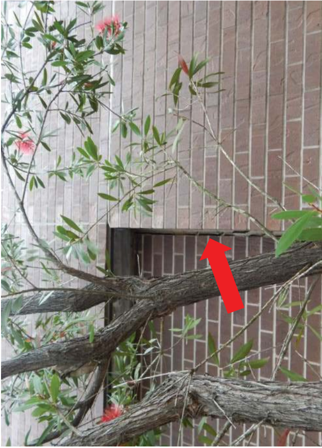
#25 Separation in caulk joint at end of inset brick panel of approximately 1/2".
