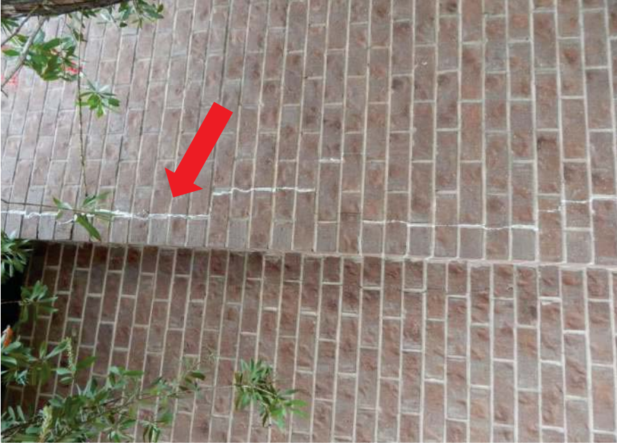
#29 Vertical crack in brick column that had been repaired.
