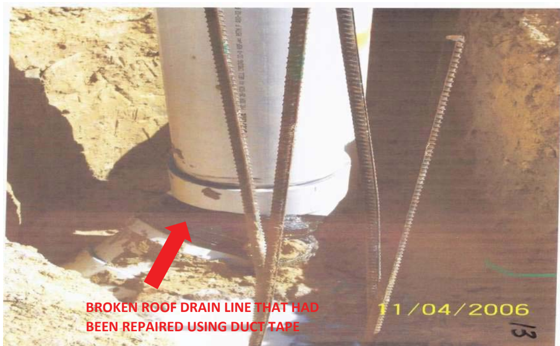
#6 Photo taken by contractor of Phase Two showing broken drain line that was repaired using duct tape
