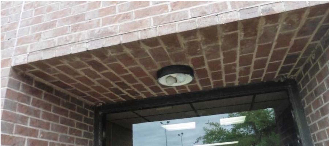
Examples of brick soffit water damage, abandoned or broken electrical
