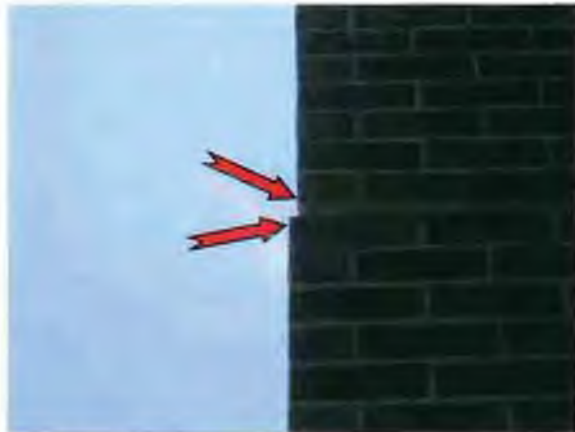
Photo #13 Lateral movement in brick veneer
