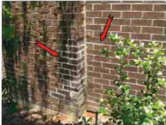
Photo #21 Masonry-mortar-joint crack
