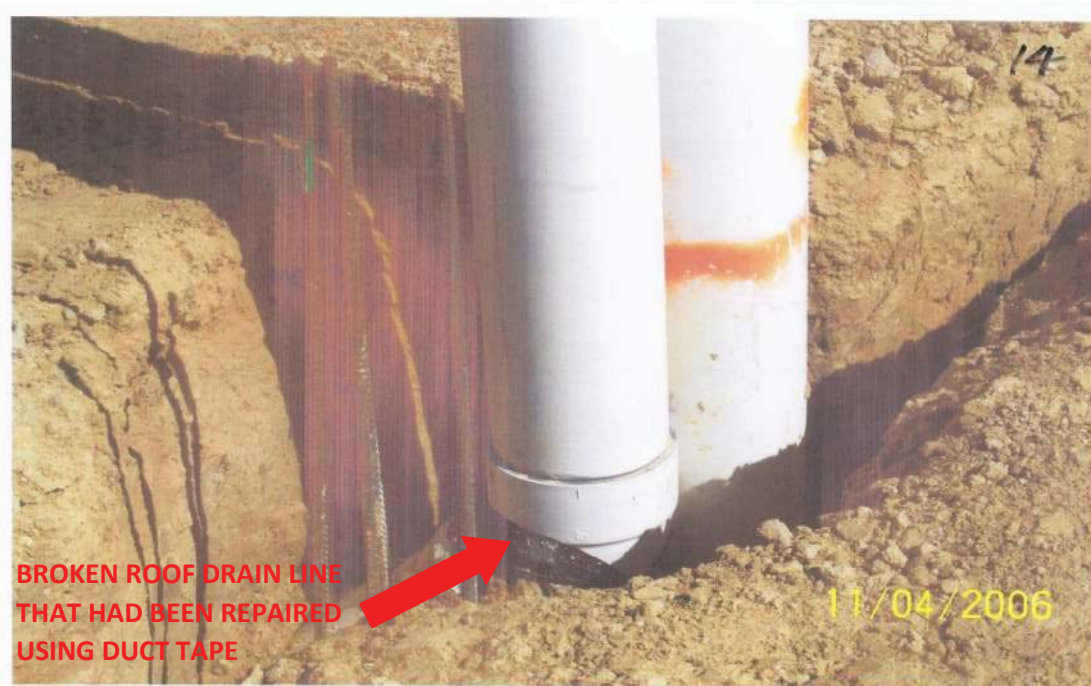
#7 Photo taken by contractor of Phase Two showing broken drain line that was repaired using duct tape and being covered with fill.
