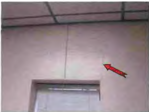
Photo #71 Crack in gypsum wallboard wall
