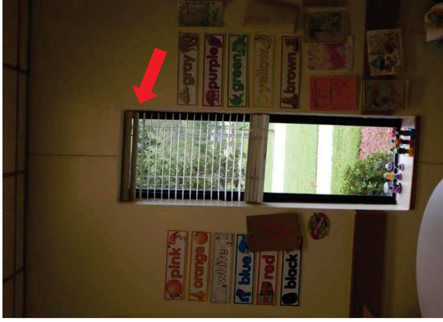
#41 Window has been tilted out of square. Photo #28 shows cracking of outside brick in this area
