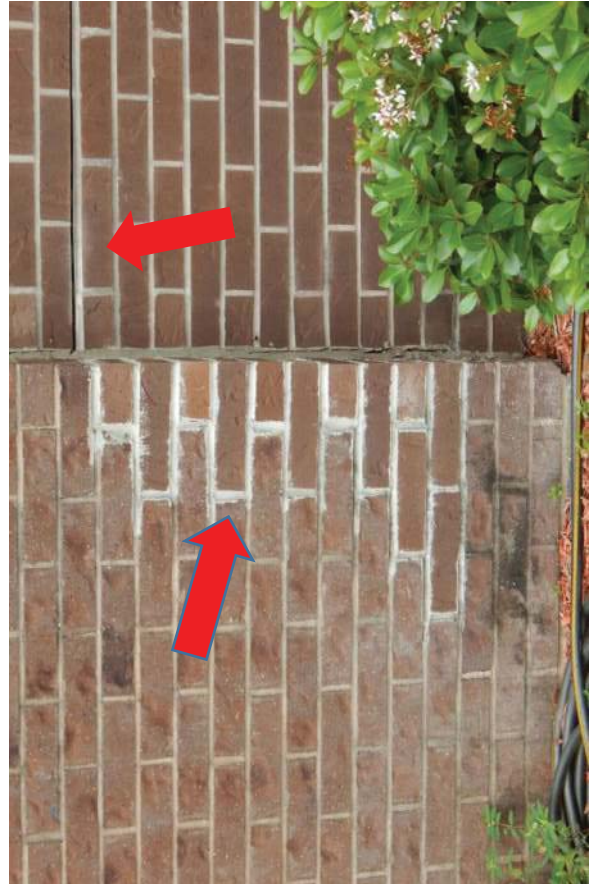
#27 Photo at connection of phase one and phase two buildings. Horizontal crack in brick in phase two. Repaired brick cracking in phase one.
