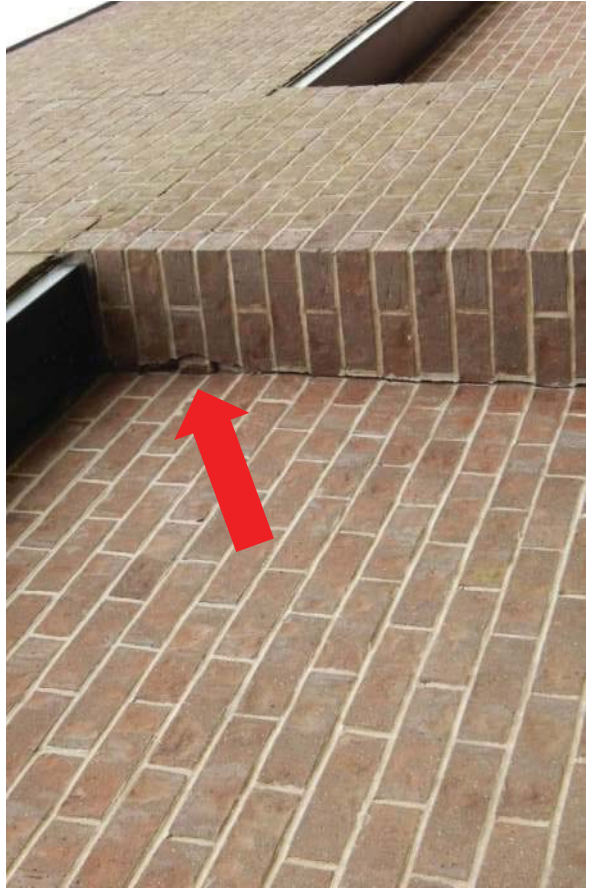
#11 Cracked brick at end of inset panel.
