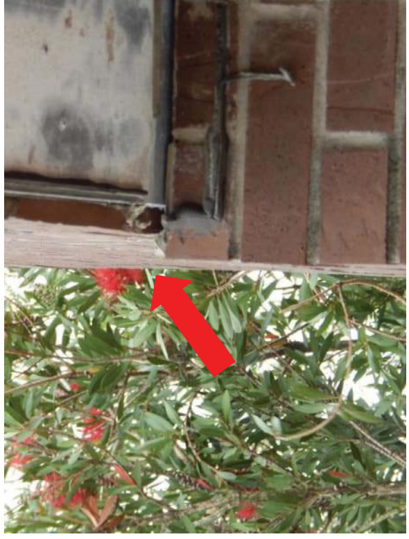
#18 Separation in caulk joint at end of inset panel. Crack does not go up in control joint above inset panel. Separation at top was measured at approximately \frac{1}{2} "
