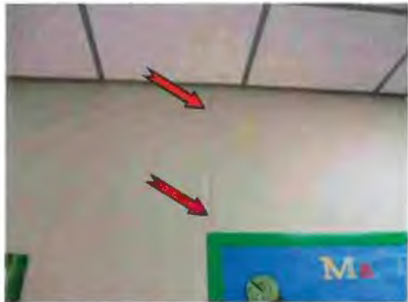
Photo #46 Crack in gypsum wallboard wall
