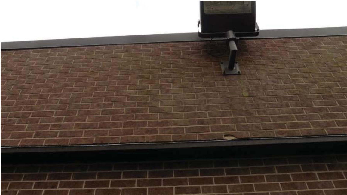
Spalled brick at an inset panel, example of existing security lighting
