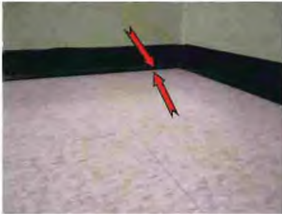
Photo #37 Separation between the baseboard and the floor
