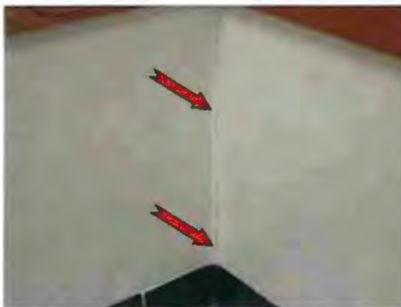
Photo #34 Crack in gypsum wallboard walls
