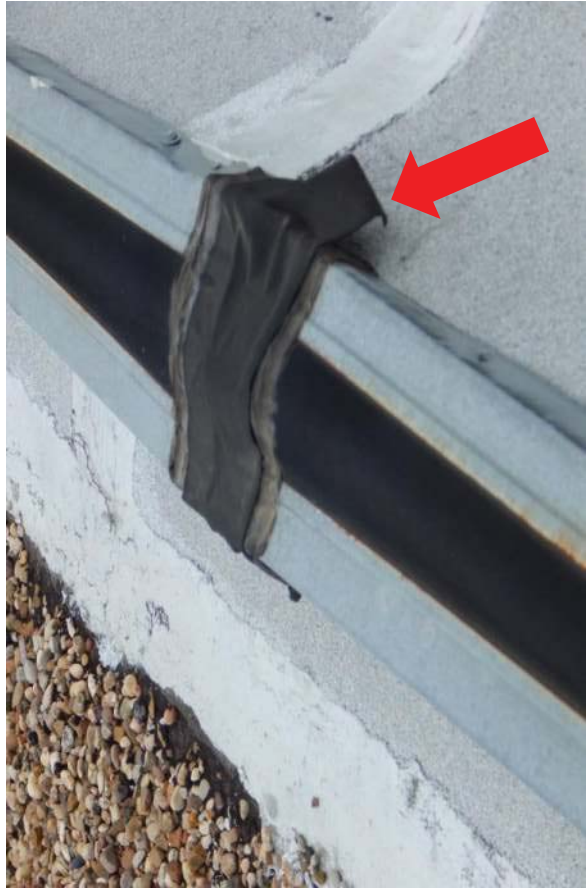
#56 Roof Expansion joint at splice where splice has come loose
