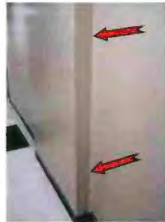
Photo #40 Crack in gypsum wallboard wall
