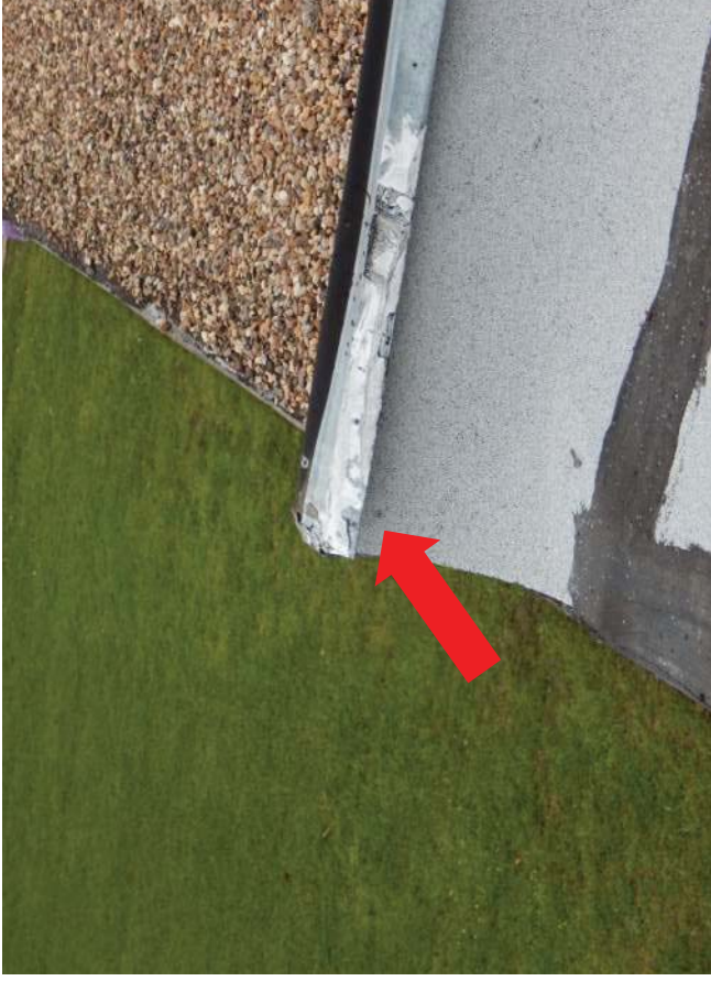
#55 End of roof expansion joint where joint is coming loose
