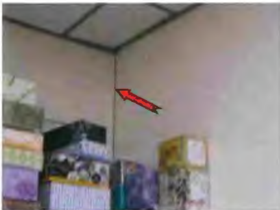
Photo #53 Separation in gypsum wallboard wall
