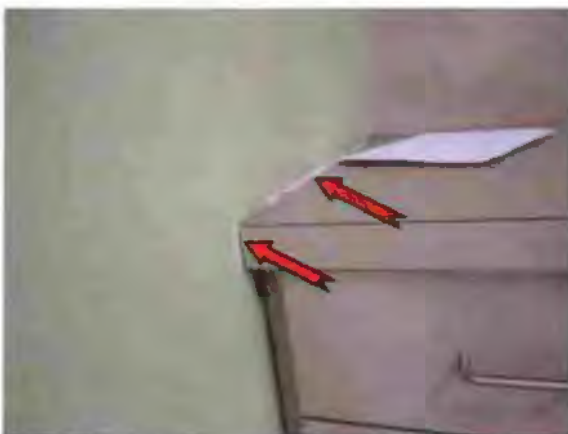
Photo #36 Separation between counter top and wall
