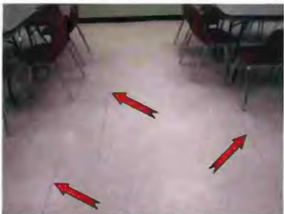
Photo #35 Separations in vinyl tile floor
