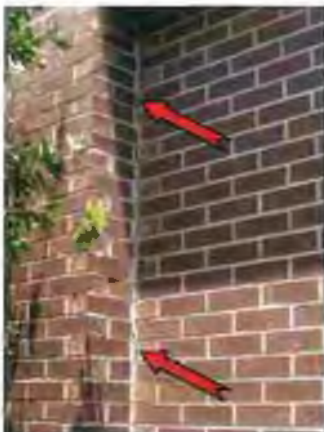
Photo #17 Separation at expansion joint
