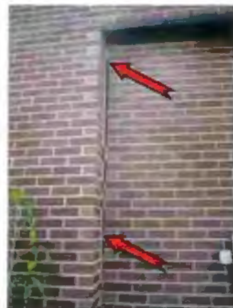
Photo #12 Separation at expansion joint
