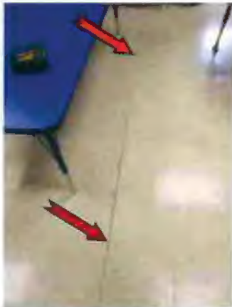
Photo #69 Separations in vinyl tile floor
