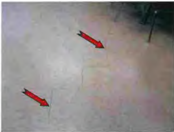
Photo #39 Separations in vinyl tile floor
