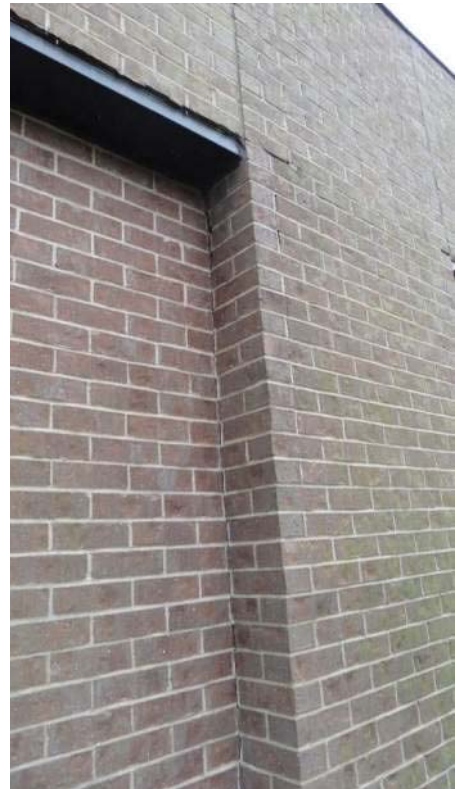
Example of missing control joints at panel inset
