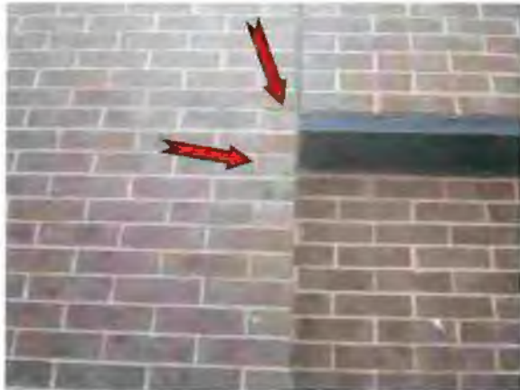
Photo #7 Masonry-mortar-joint crack
