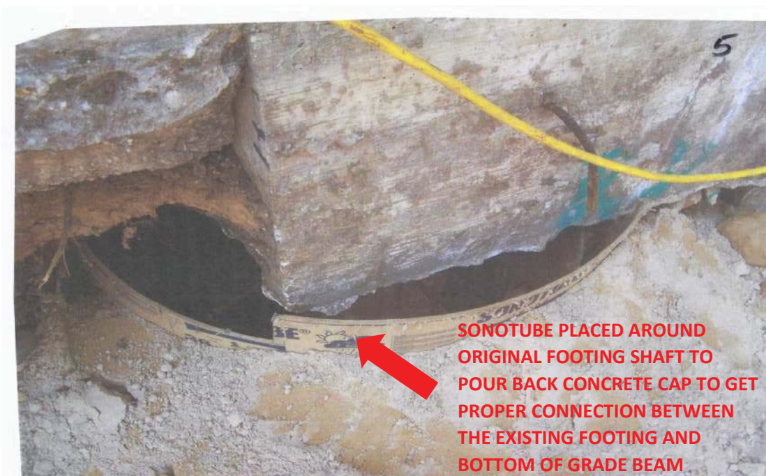
#4 Photo taken by contractor of Phase Two showing how concrete cap was being poured between existing footing and grade beam
