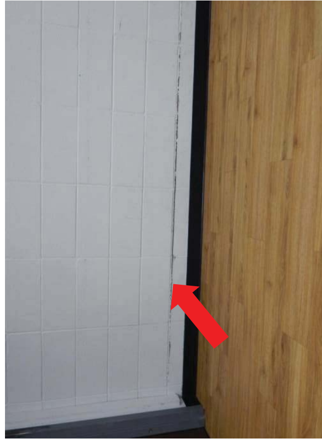
#46 Horizontal crack at base of CMU wall
