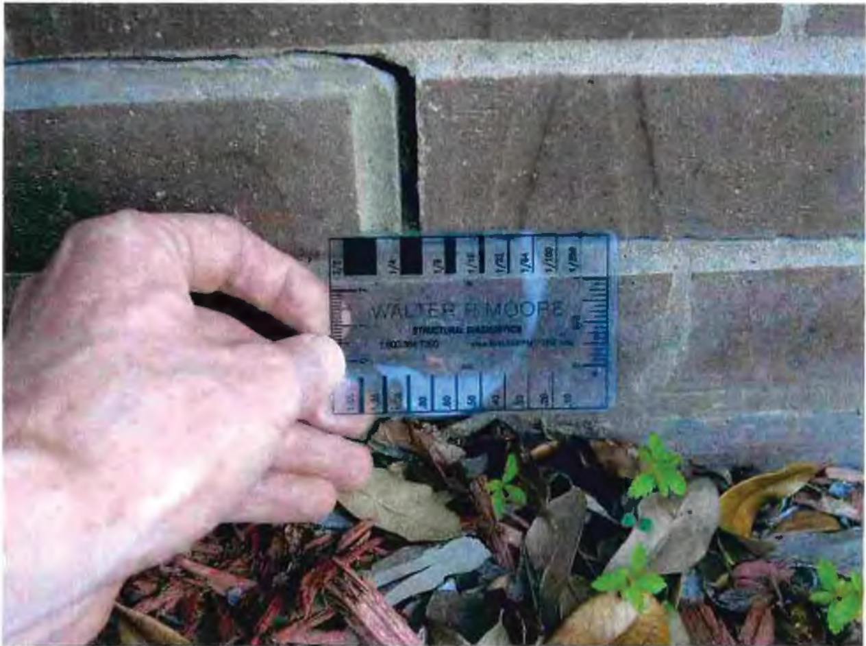
Photo 4. Exterior façade crack (in addition) near original building.
