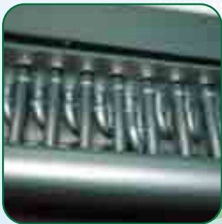
New Equipment Coils Treated with EGuard DCC Green
