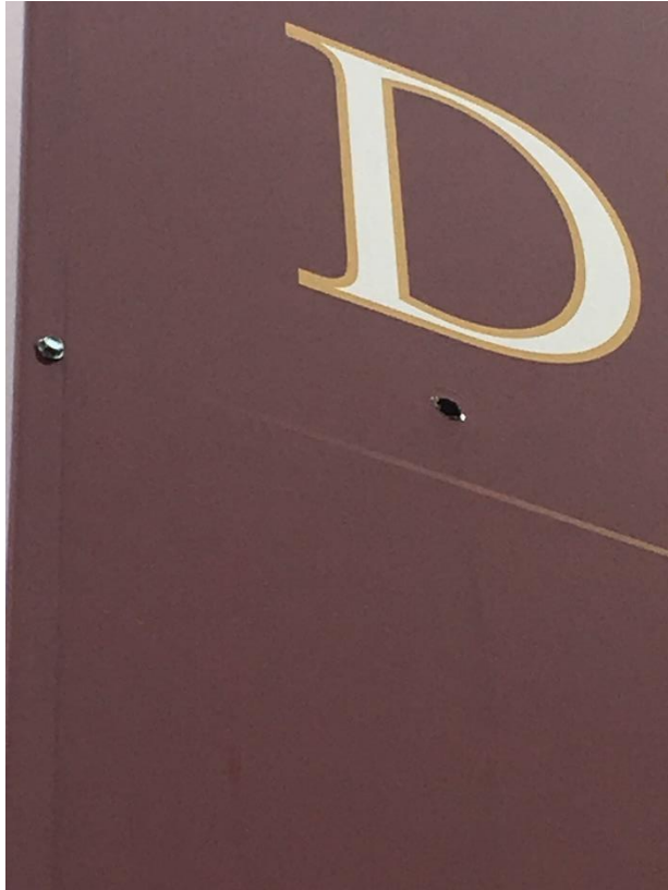
Example 9: Bolts falling out of signs and leaving holes.
