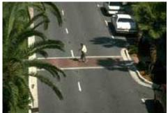
Figure 34. Curb extensions at midblock locations reduce crossing distance for pedestrians.
