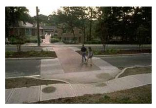
Figure 36. Raised crosswalks can control vehicle speeds on local streets at pedestrian crossings.
